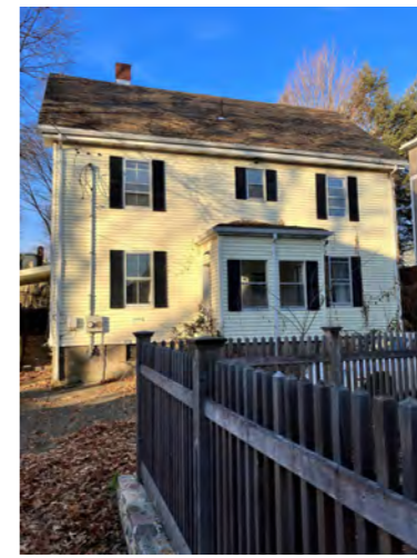
92 Holworthy St East Elevation
