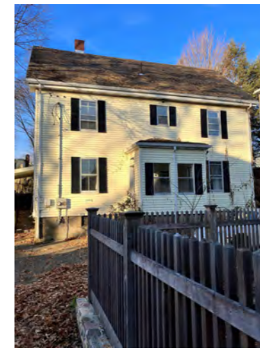
92 Holworthy St East Elevation
