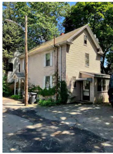
4 Holworthy Terrace North & West Elevations
