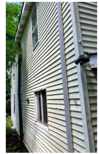
92 Holworthy St West Elevation
