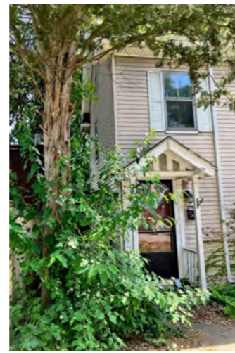
4 Holworthy Terrace Entry & East Elevation
