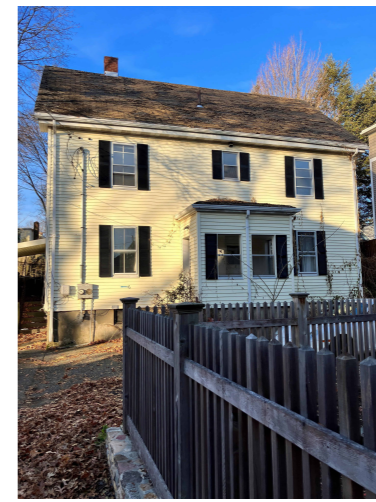
92 Holworthy St East Elevation
