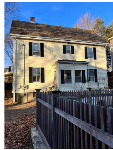
92 Holworthy St East Elevation
