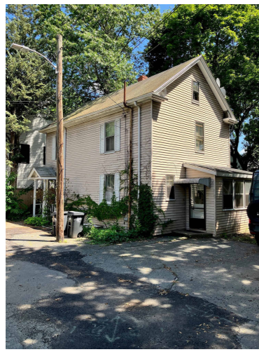
4 Holworthy Terrace North & West Elevations
