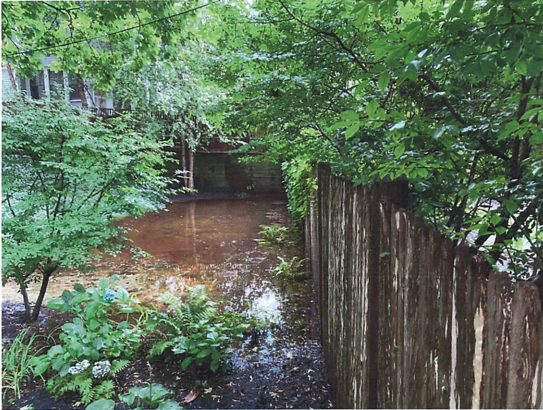
Image 2. Backyard of 50 Concord after heavy rain in September 2021.
