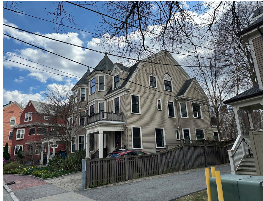
VIEW 2 - West Elevation (50 Wendell St)
