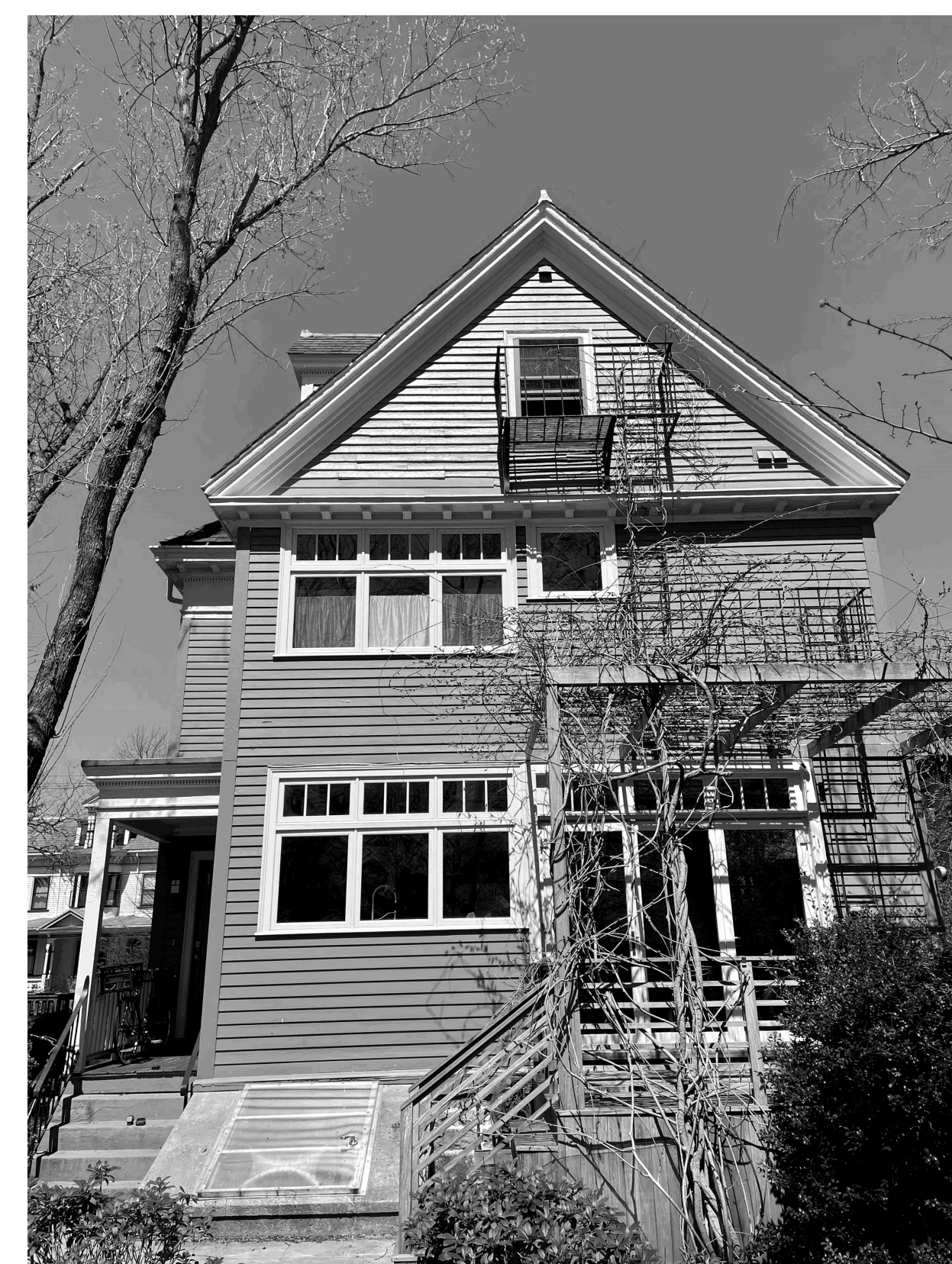
54 GARFIELD STREET - SOUTH VIEW FROM BACKYARD
