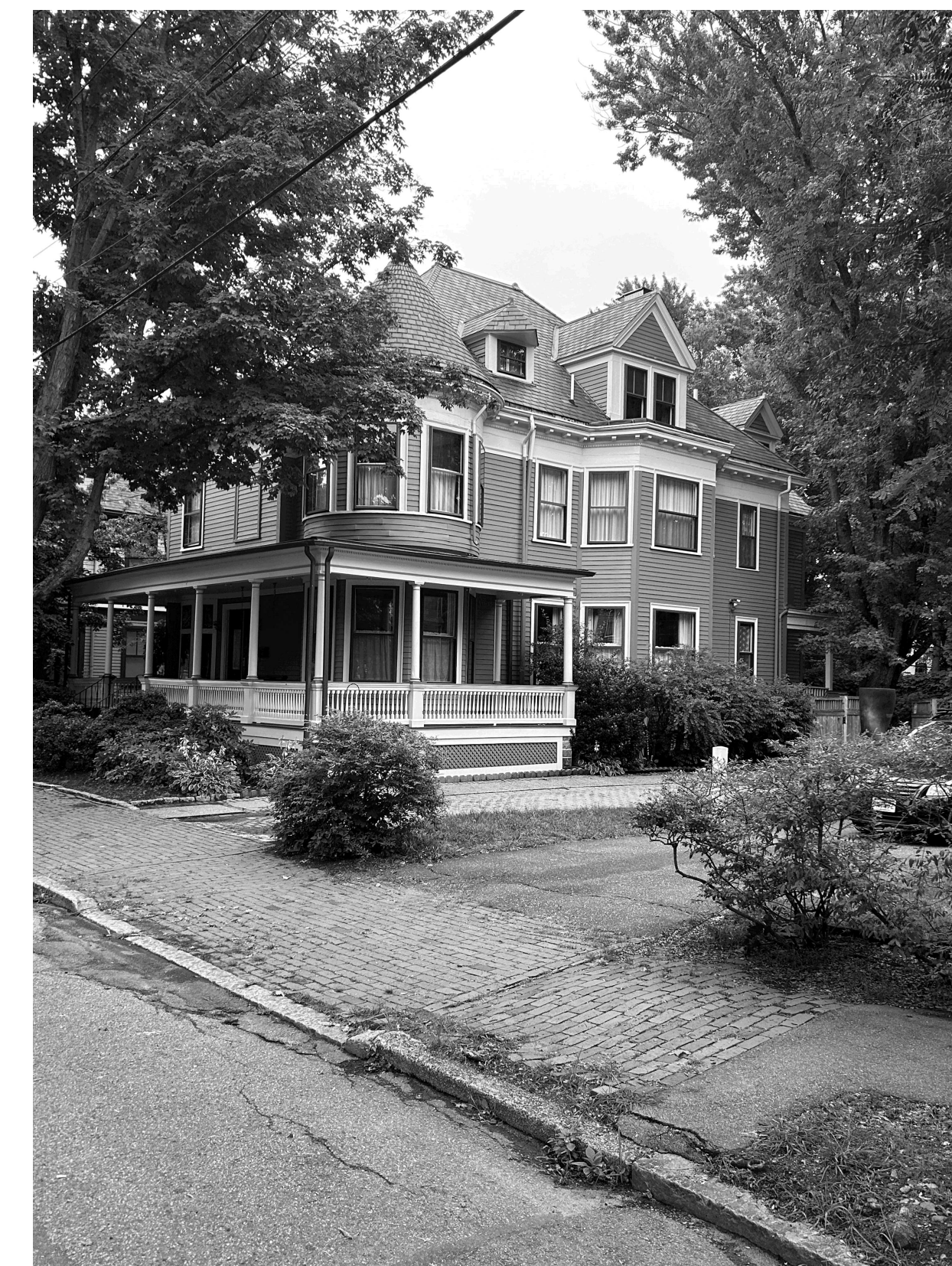
54 GARFIELD STREET - NORTHWEST VIEW FROM STREET
