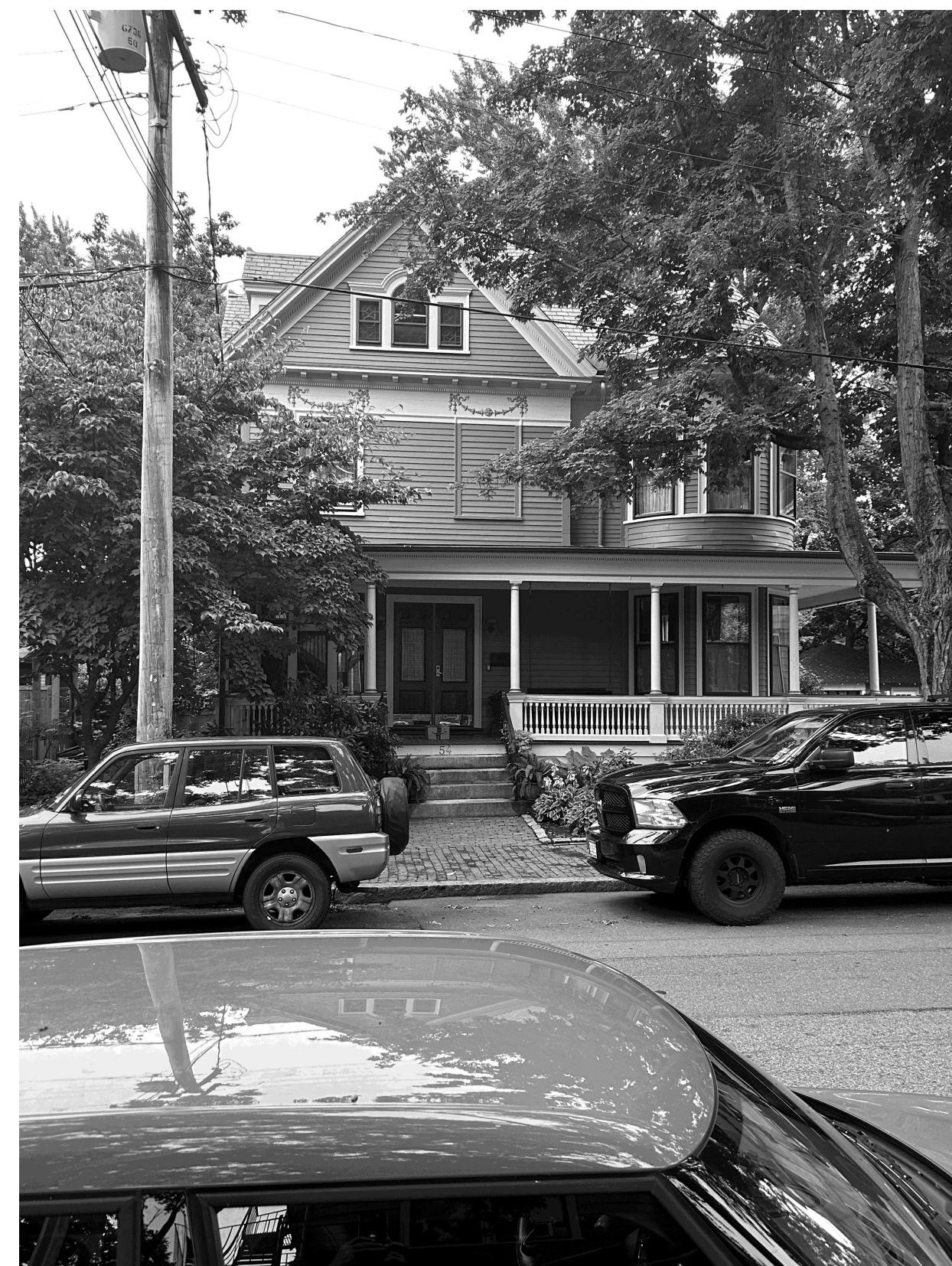
54 GARFIELD STREET - NORTH VIEW FROM ACROSS THE STREET
