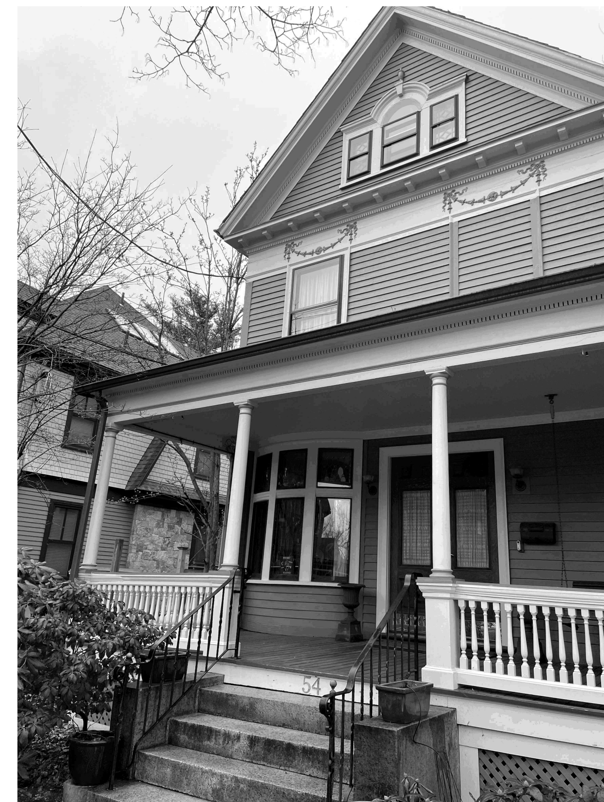
54 GARFIELD STREET - NORTH VIEW FROM SIDEWALK
