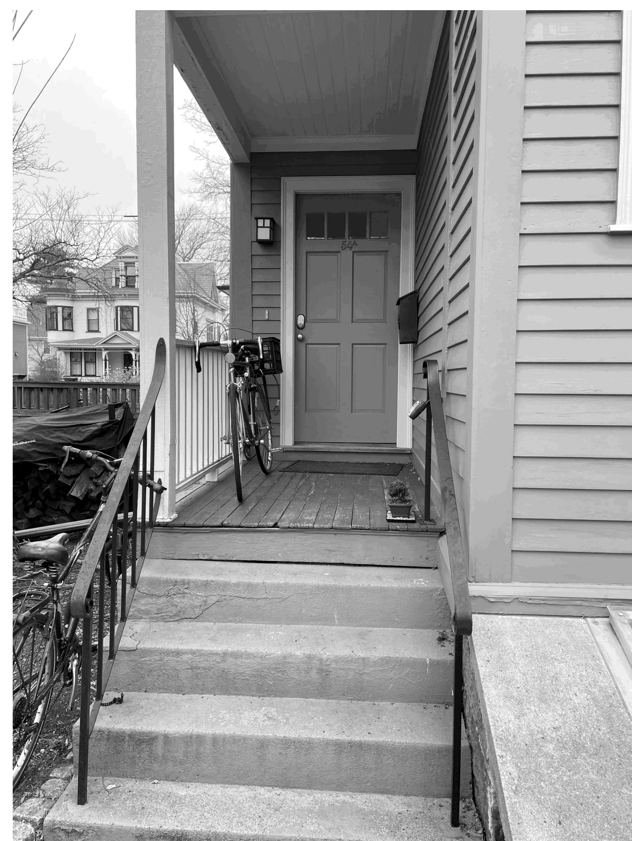
54 GARFIELD STREET - SOUTH VIEW OF EXISTING PORCH FROM BACKYARD
