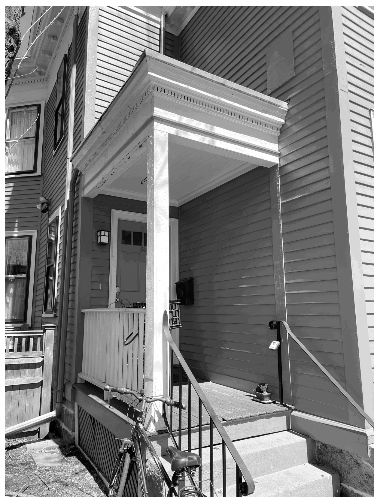
54 GARFIELD STREET - SOUTHWEST VIEW OF EXISTING PORCH FROM BACKYARD
