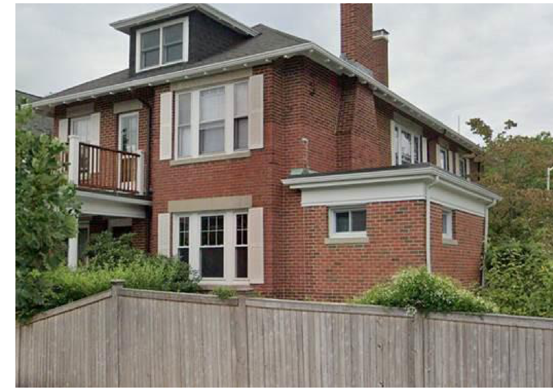
AREA OF OFFICE ADDITION (HURON AVENUE)
