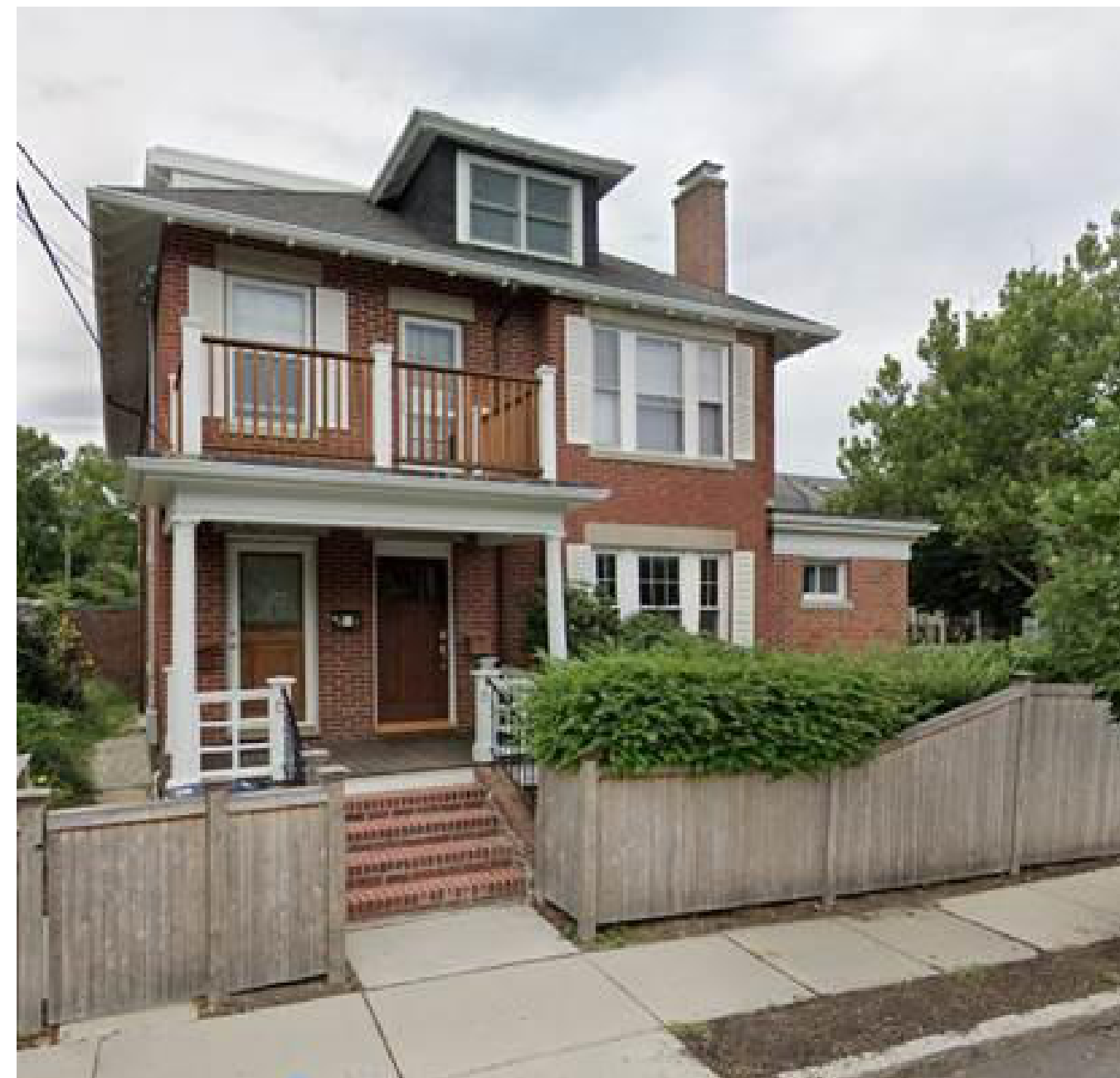
AREA OF BEDROOM ADDITION (RESERVOIR STREET)
