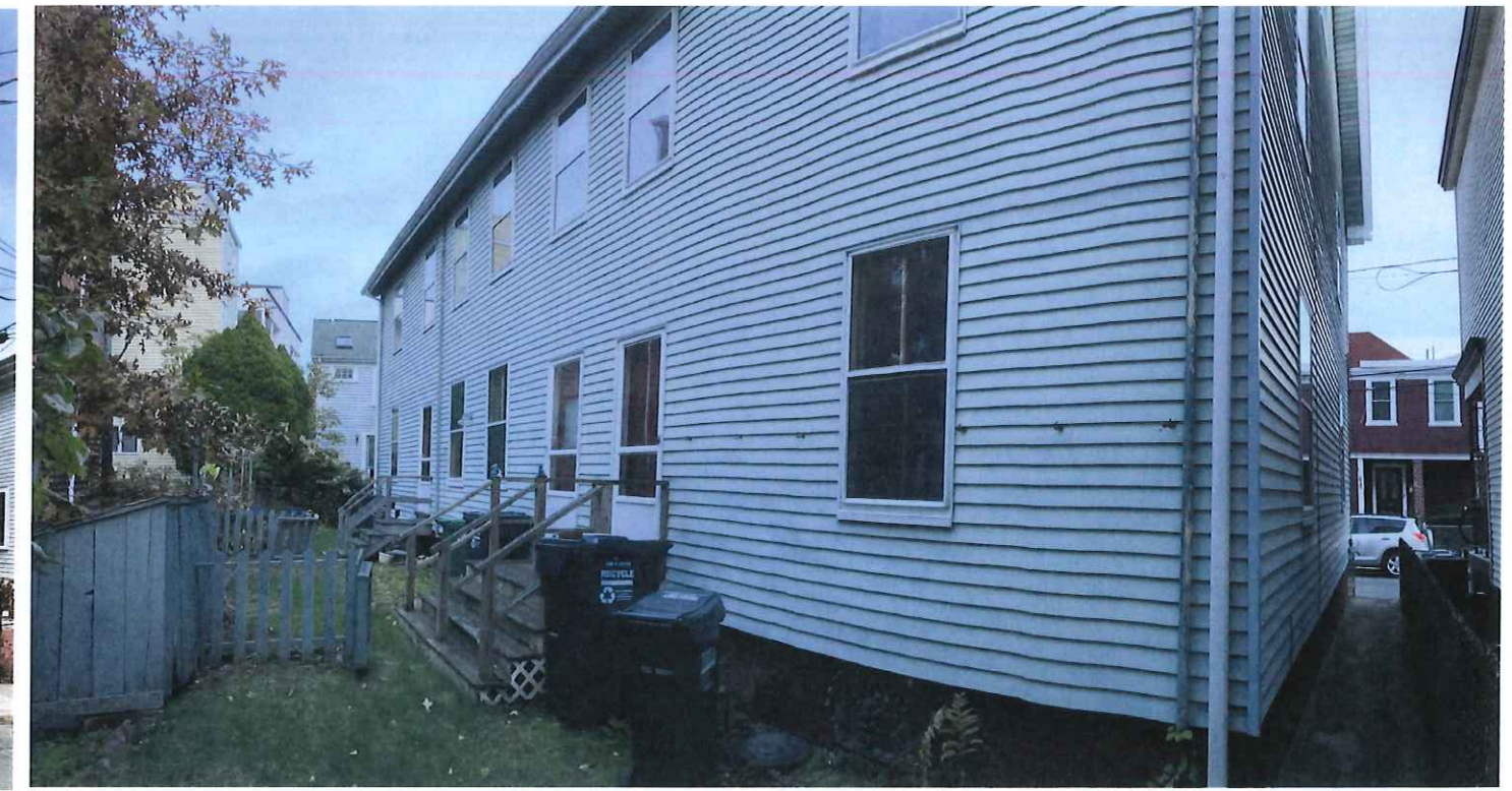
Rear Yard and Facade
