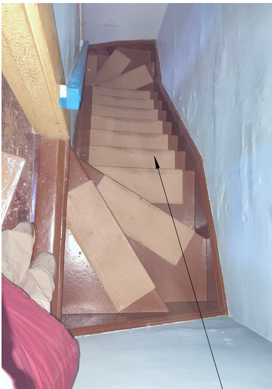
Stairs to Attic Floor
