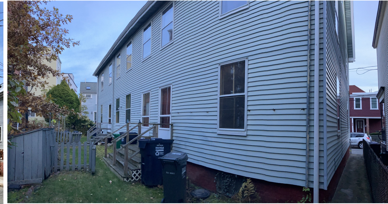
Rear Yard and Facade
