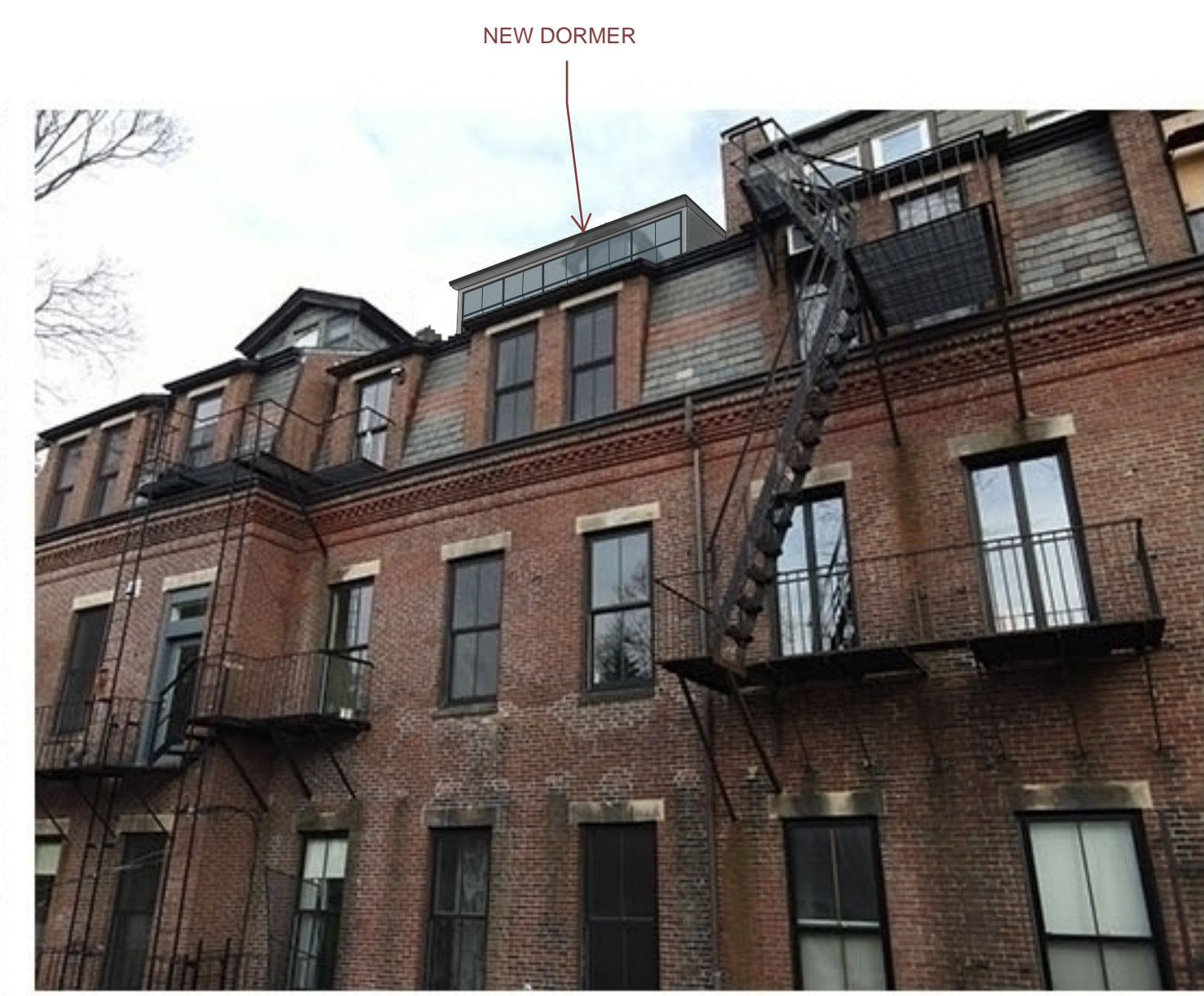
6 - REAR YARD VIEW UP WITH DORMER / TERRACE
