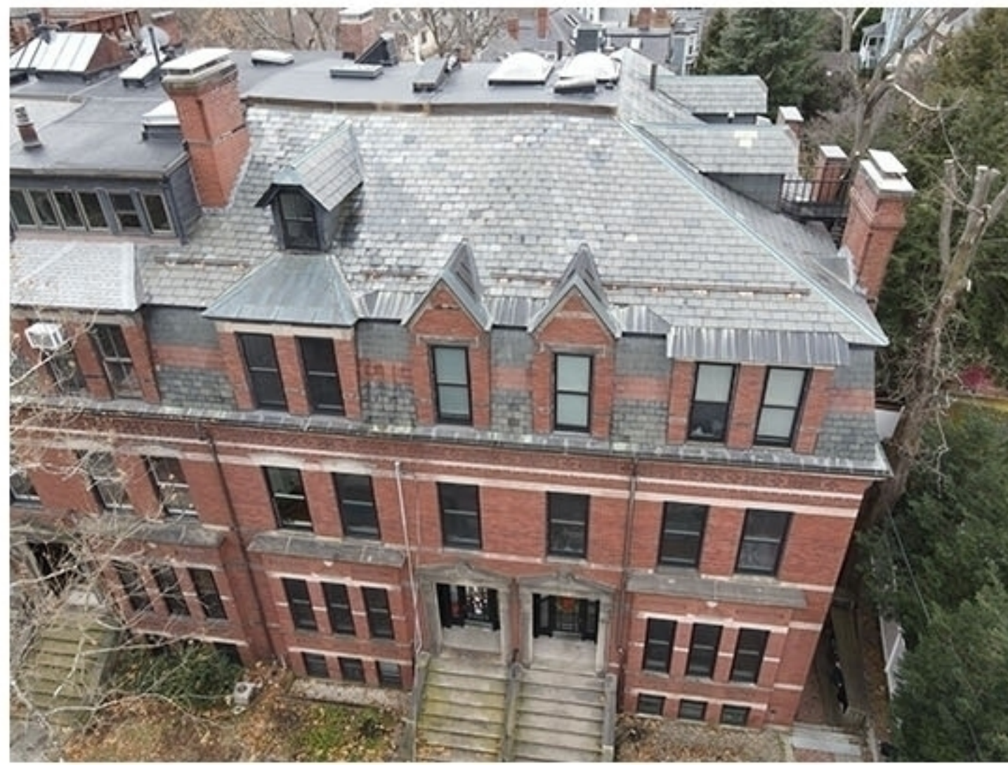
2 - VIEW FROM FRONT YARD, EXISTING
