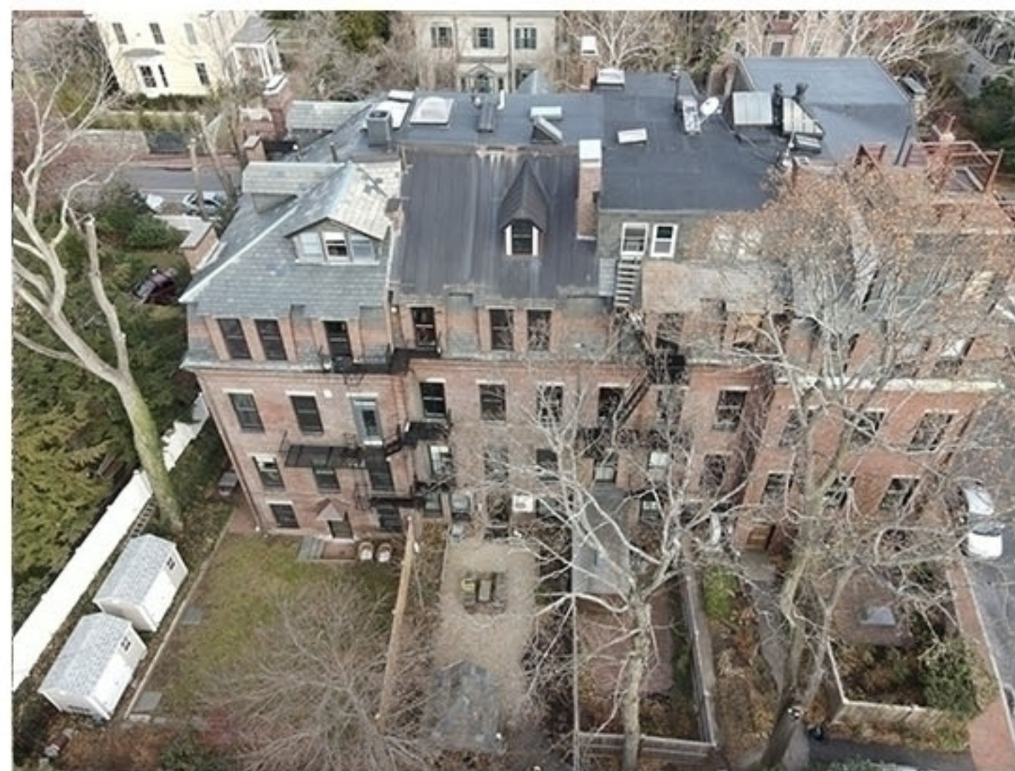
2 - REAR YARD WEST VIEW, EXISTING
