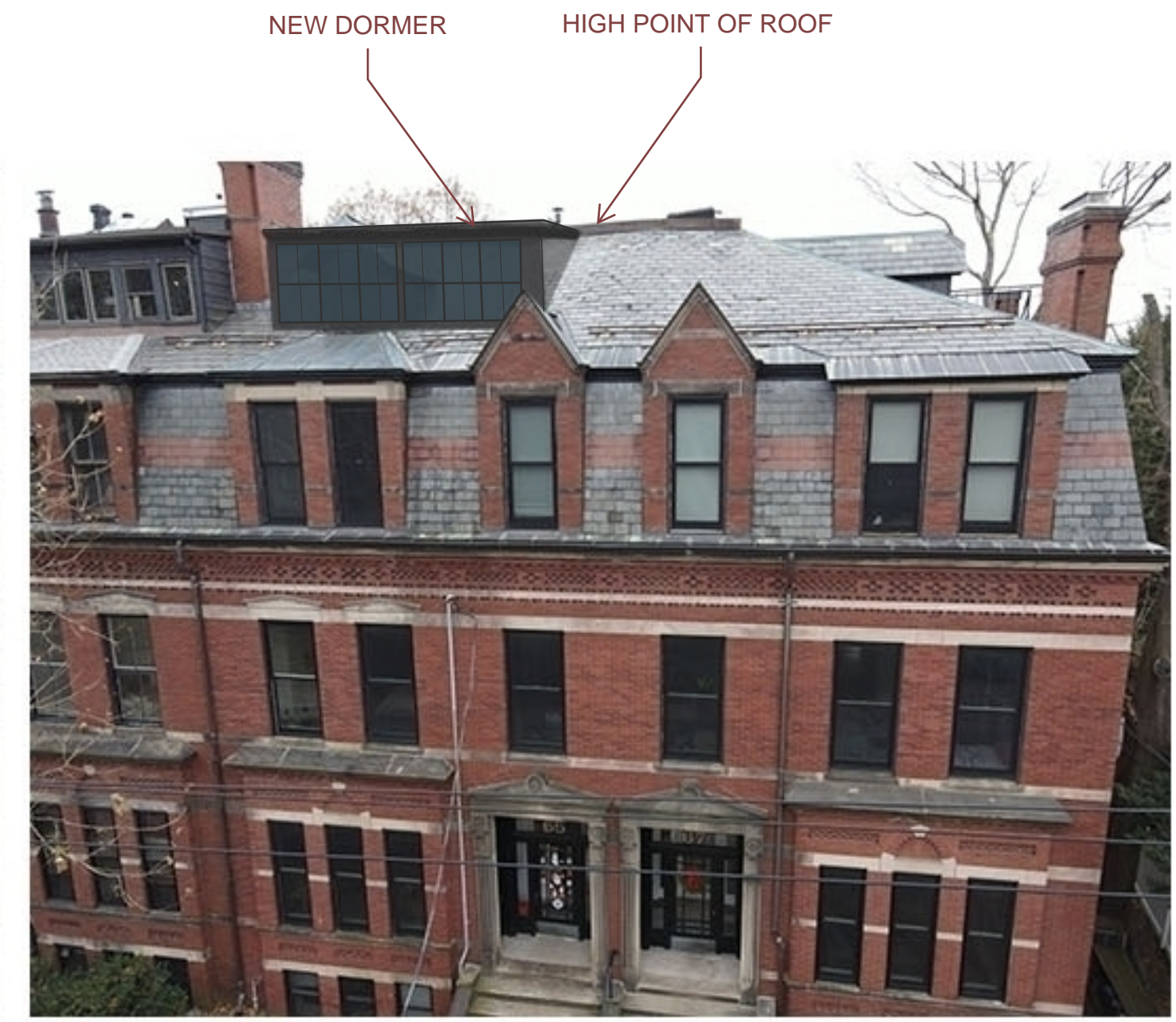
6 - VIEW UP TO ROOF WITH DORMER
