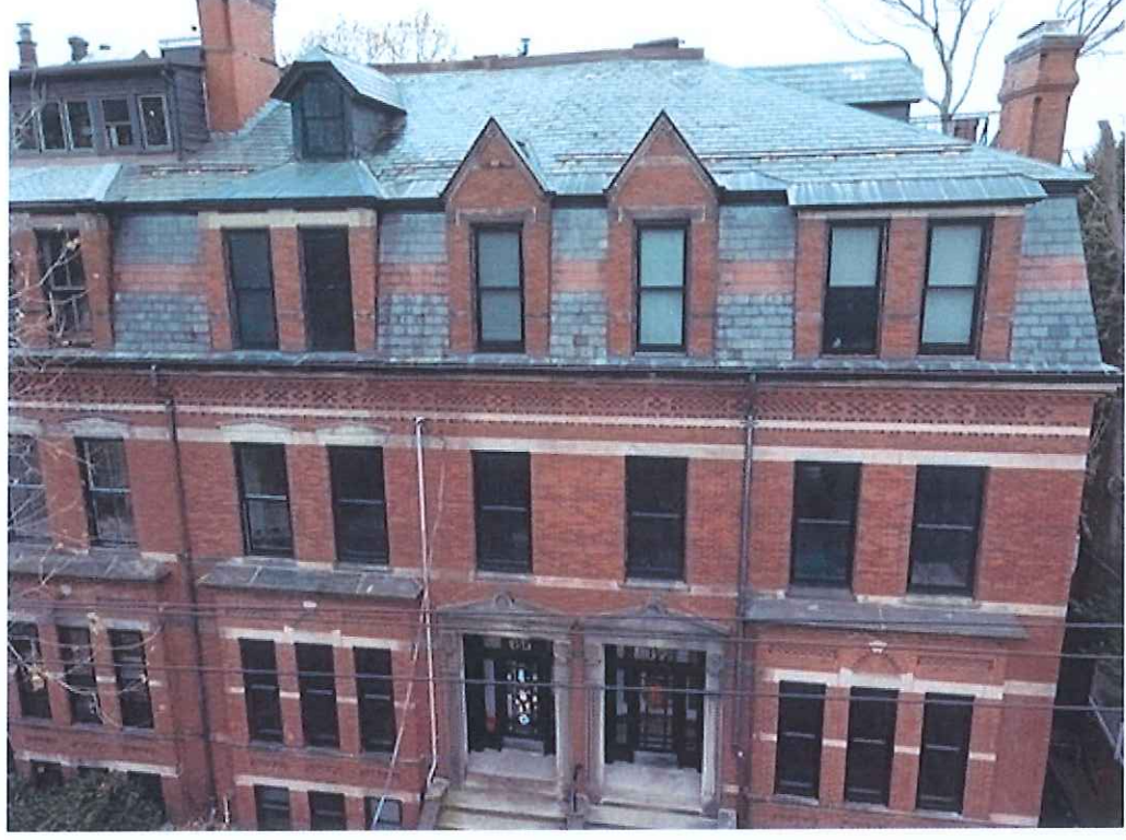
3 - VIEW UP TO ROOF, EXISTING
