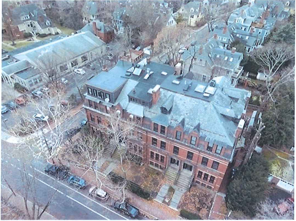
1 - VIEW FROM NORTHEAST CORNER, EXISTING
