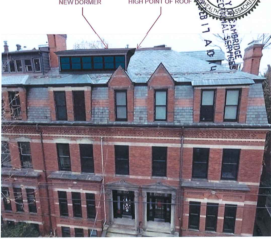
6 - VIEW UP TO ROOF WITH DORMER
