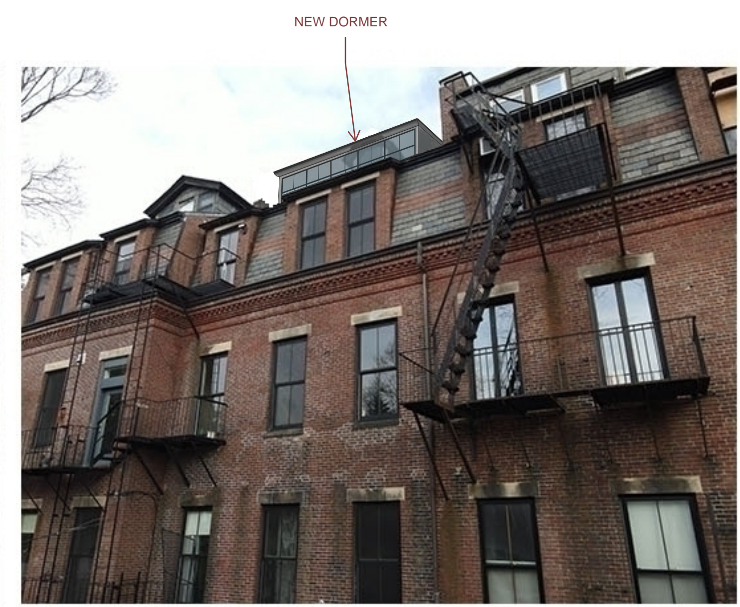
6 - REAR YARD VIEW UP WITH DORMER / TERRACE
