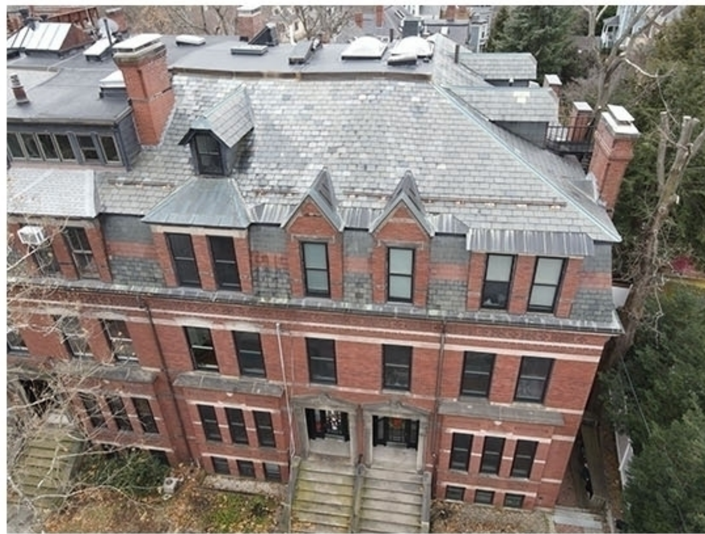
2 - VIEW FROM FRONT YARD, EXISTING
