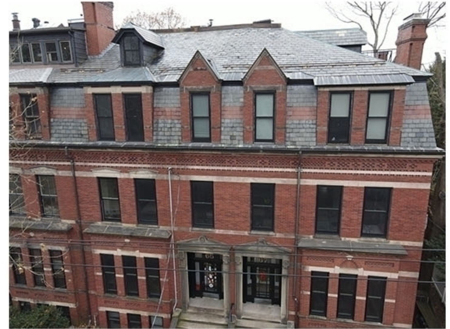
3 - VIEW UP TO ROOF, EXISTING
