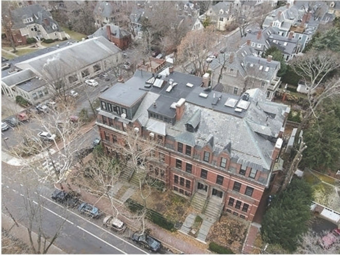
1 - VIEW FROM NORTHEAST CORNER, EXISTING
