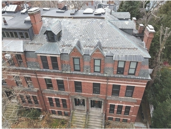
2 - VIEW FROM FRONT YARD, EXISTING
