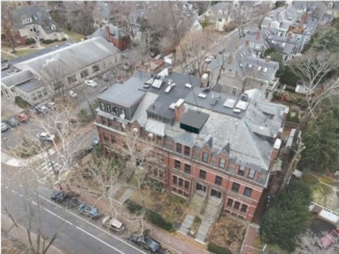
4 - VIEW FROM NORTHEAST CORNER WITH DORMER
