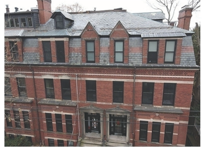
3 - VIEW UP TO ROOF, EXISTING
