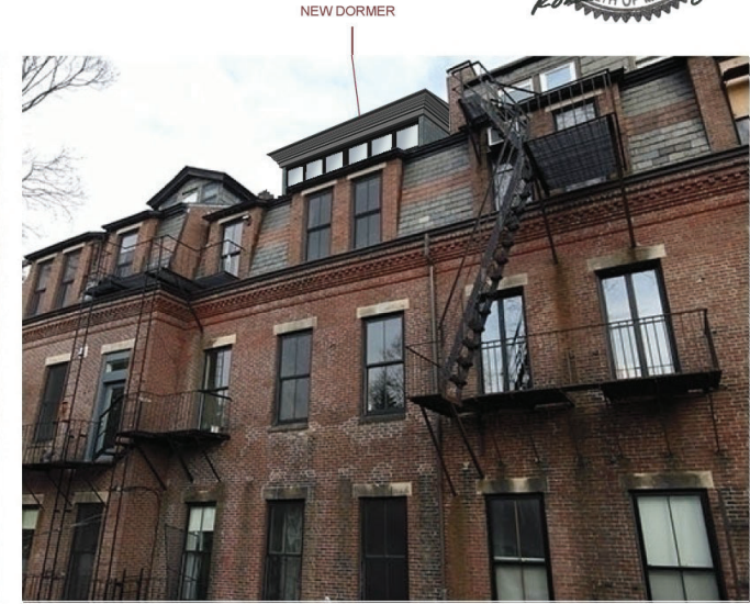
6 - REAR YARD VIEW UP WITH DORMER / TERRACE
