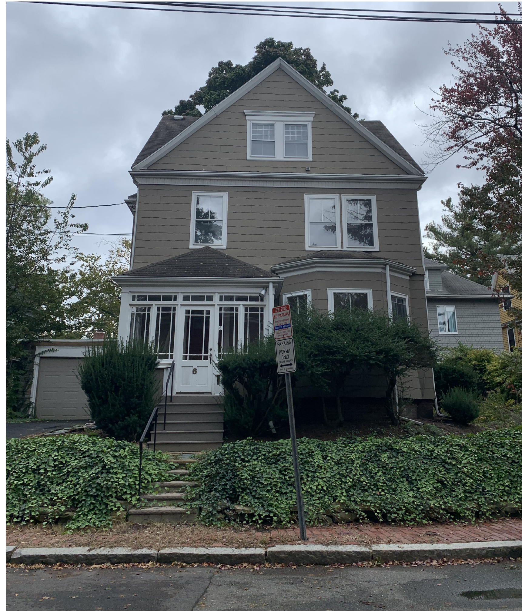
VIEW FROM SIDEWALK LOOKING AT NORTH EXTERIOR ELEVATION
