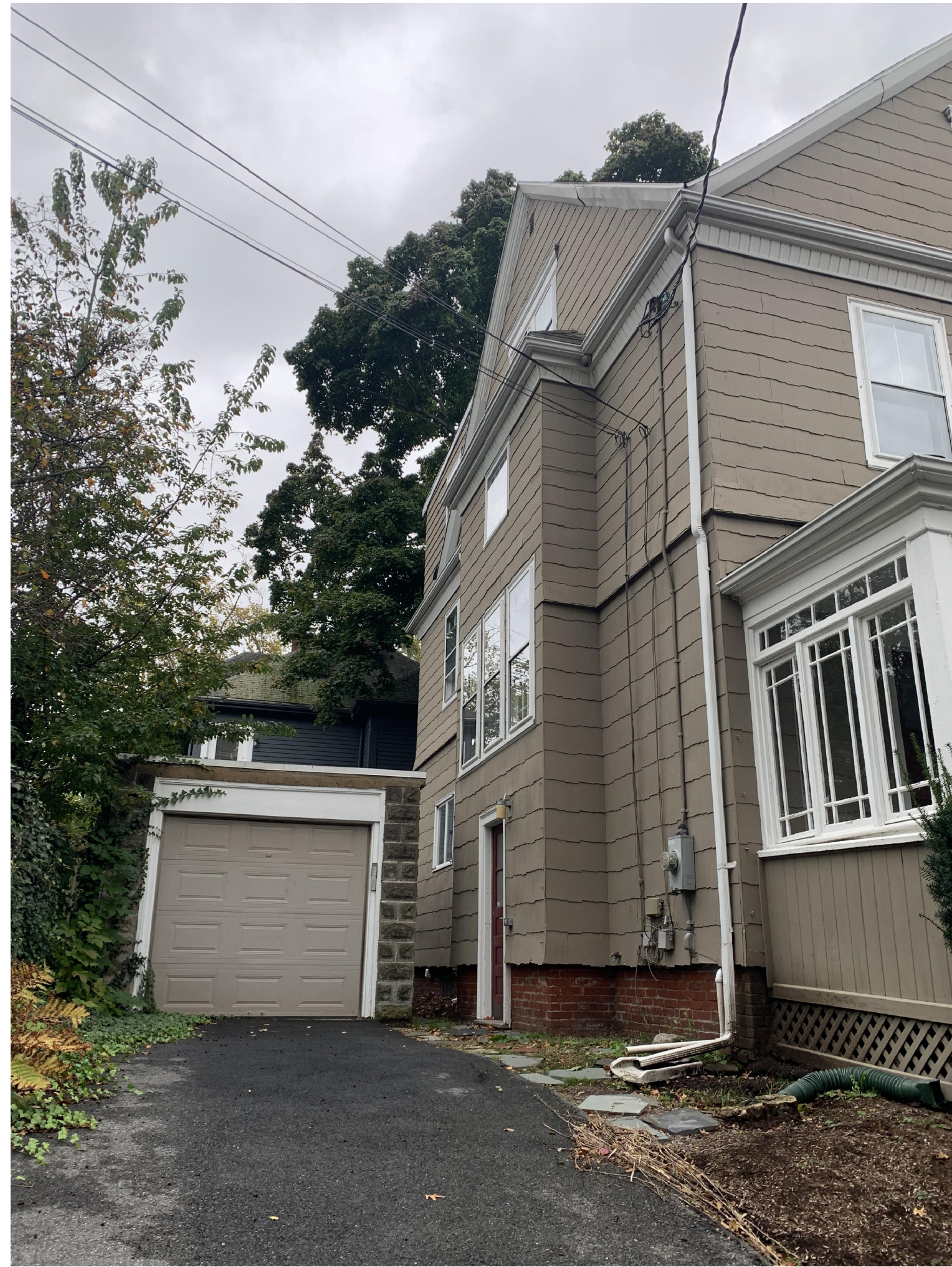
VIEW FROM SIDEWALK LOOKING SOUTH AT NORTH ELEVATION OF GARAGE
