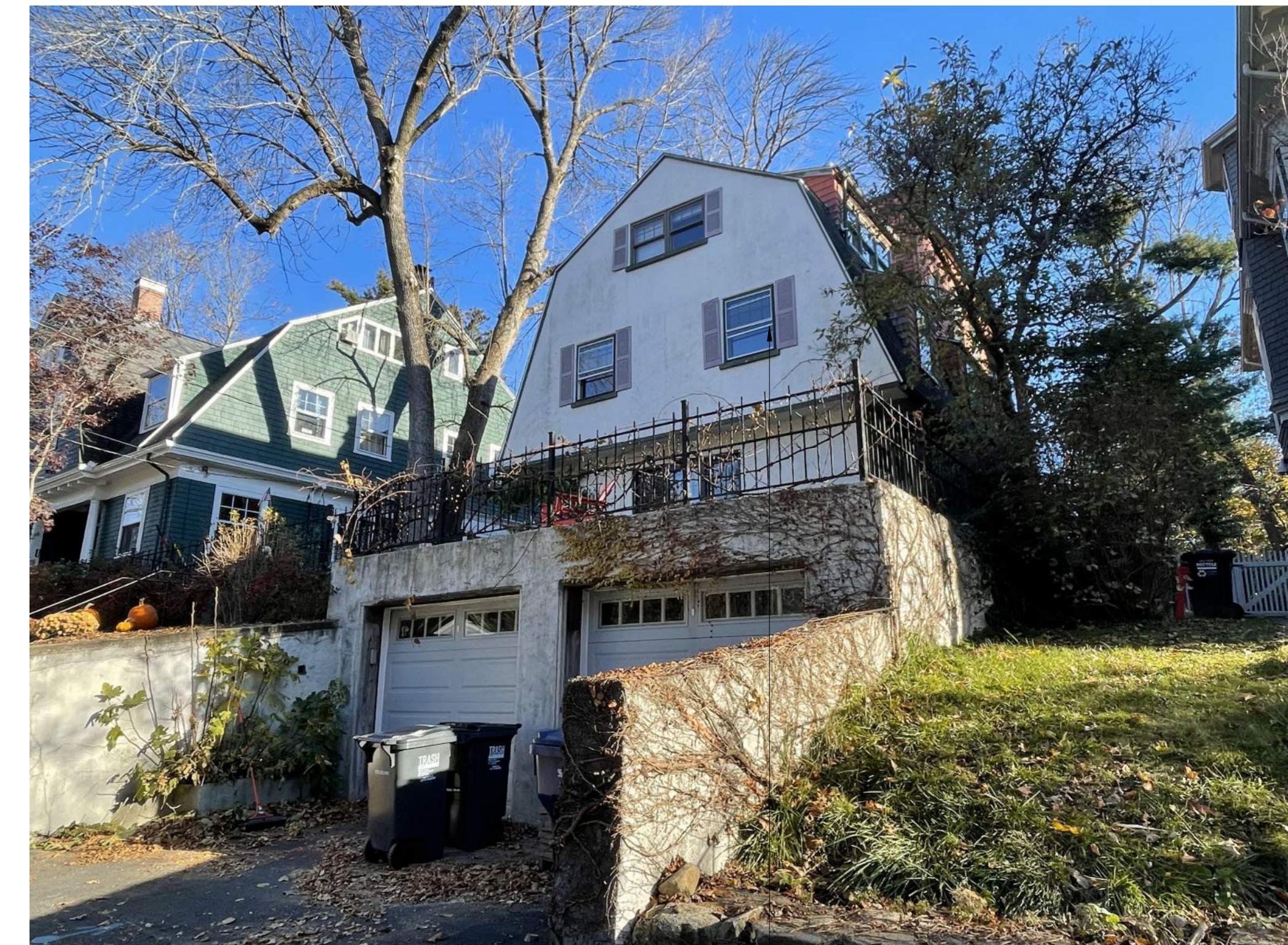
EXISTING WINDOWS 6 LITES OVER 1, TRIPLE TRACK STORM WINS
