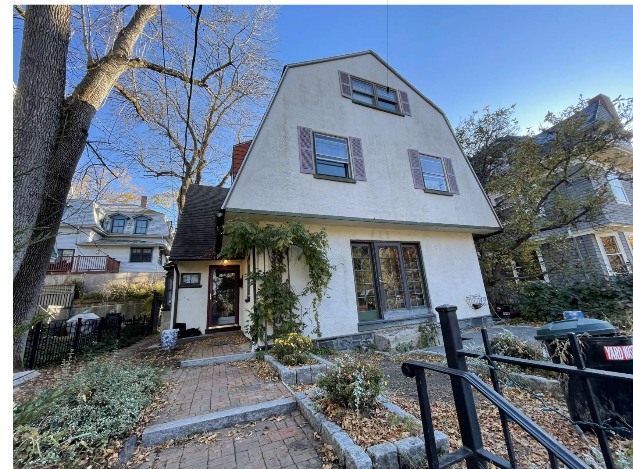
EXISTING WINDOWS 6 LITES OVER 1, TRIPLE TRACK STORM WINS
