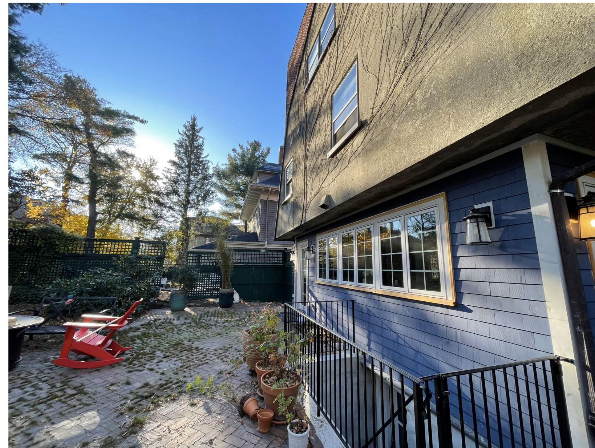
RECENTLY INSTALLED REAR FACING MARVIN WINDOWS
