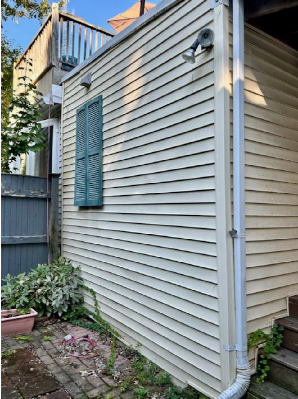
VIEW OF REAR ELEVATION OF ONE STORY ADDITION
