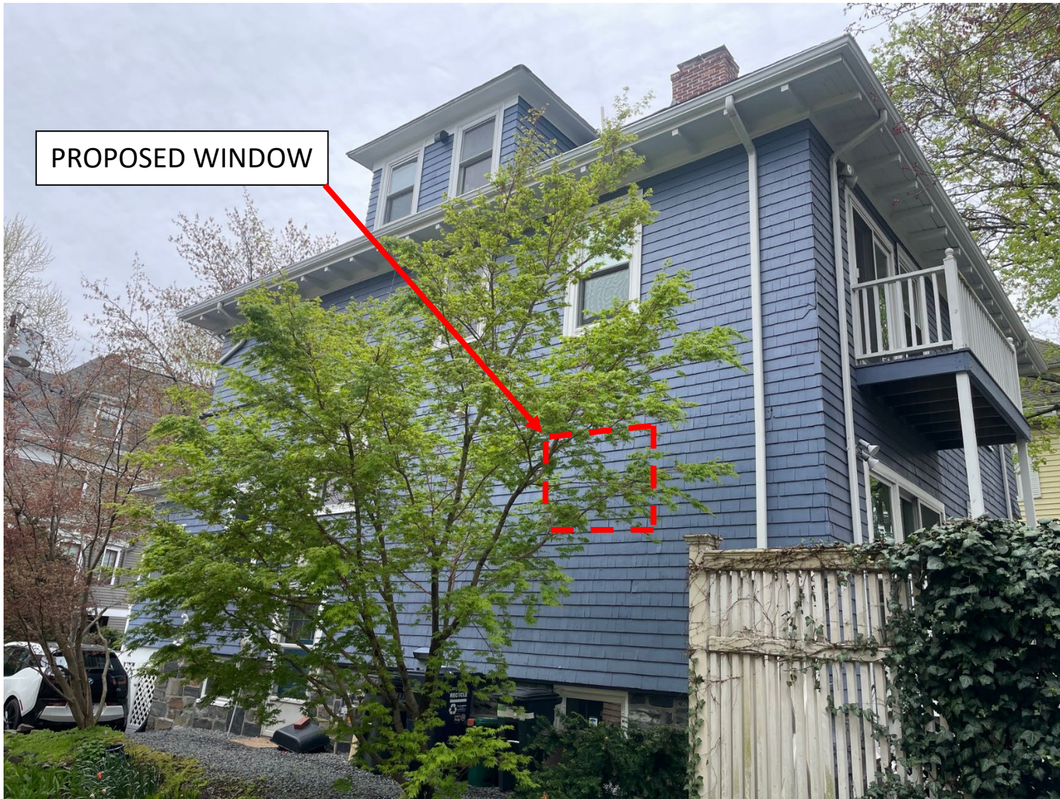
8 WHITTIER STREET – NORTH WALL (SIDE)
