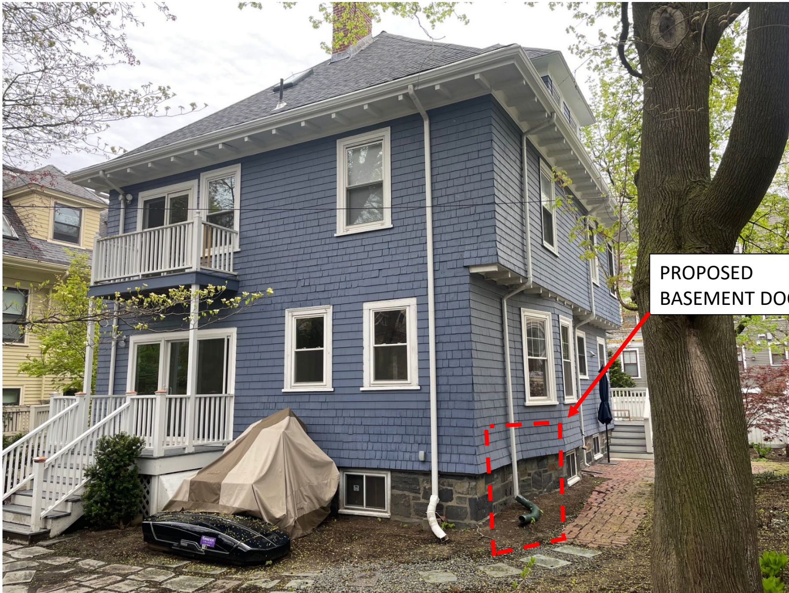
8 WHITTIER STREET – WEST & SOUTH WALLS (REAR & SIDE)
