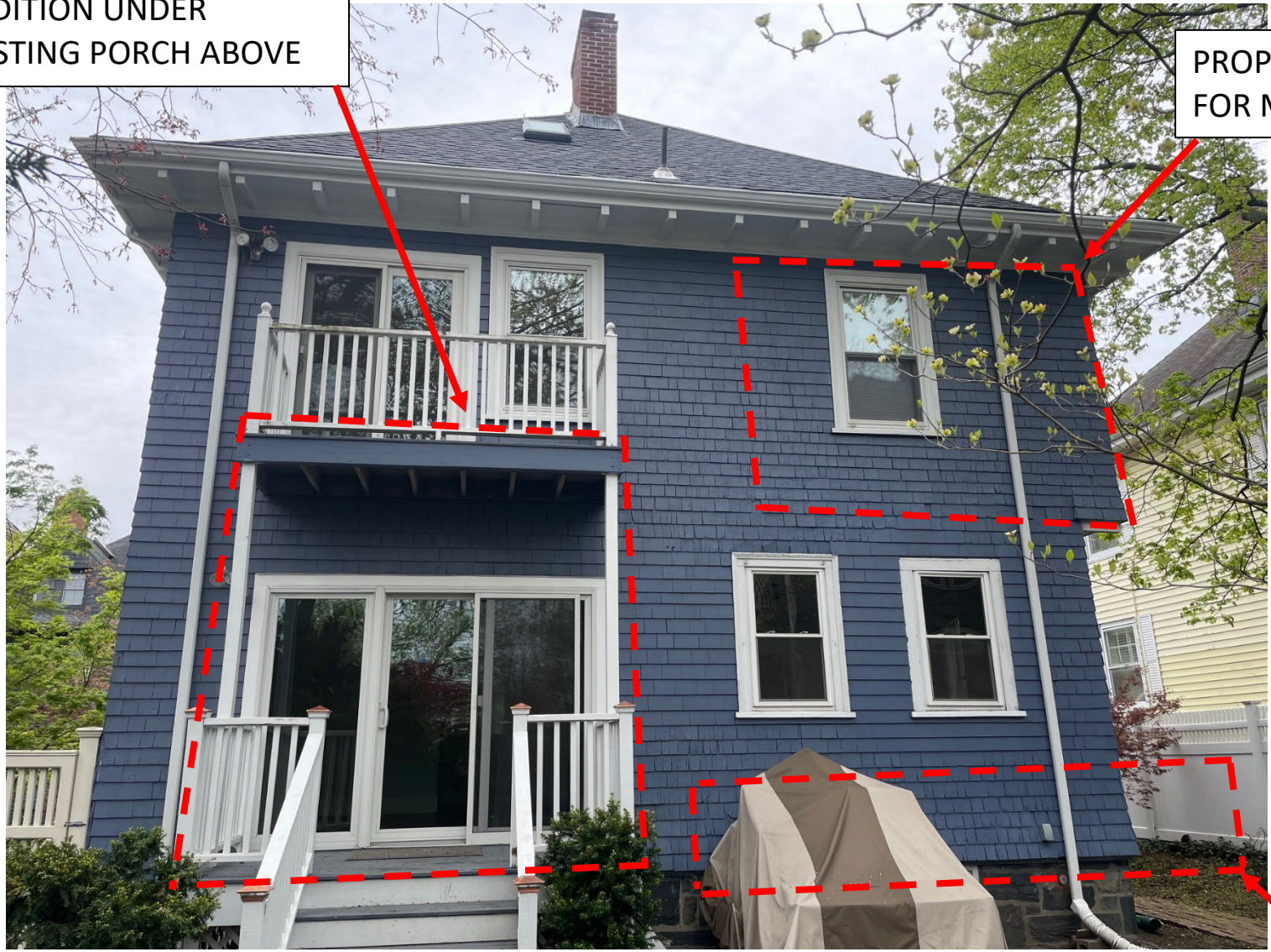
8 WHITTIER STREET – WEST WALL (REAR)
