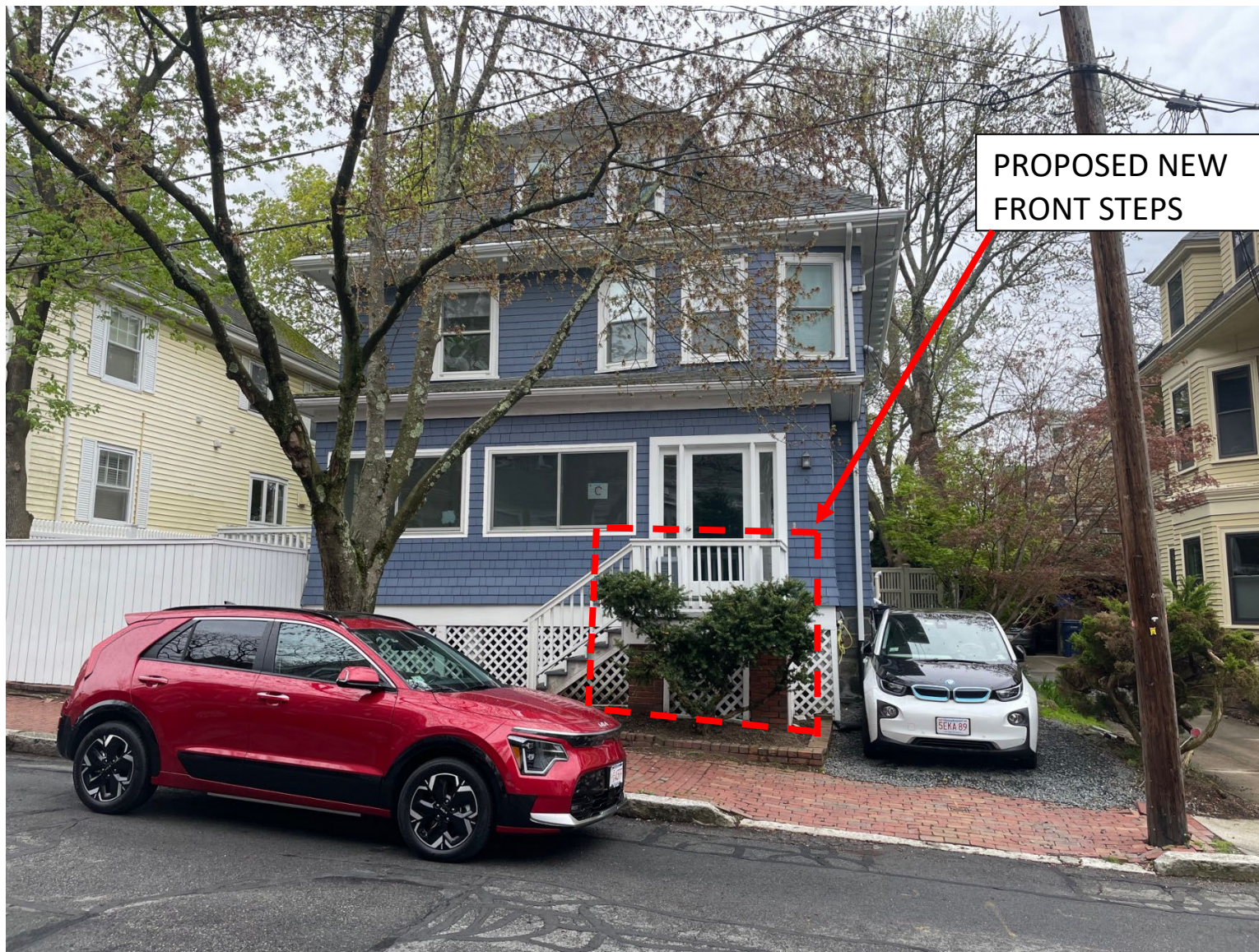
8 WHITTIER STREET – EAST WALL (FRONT)
