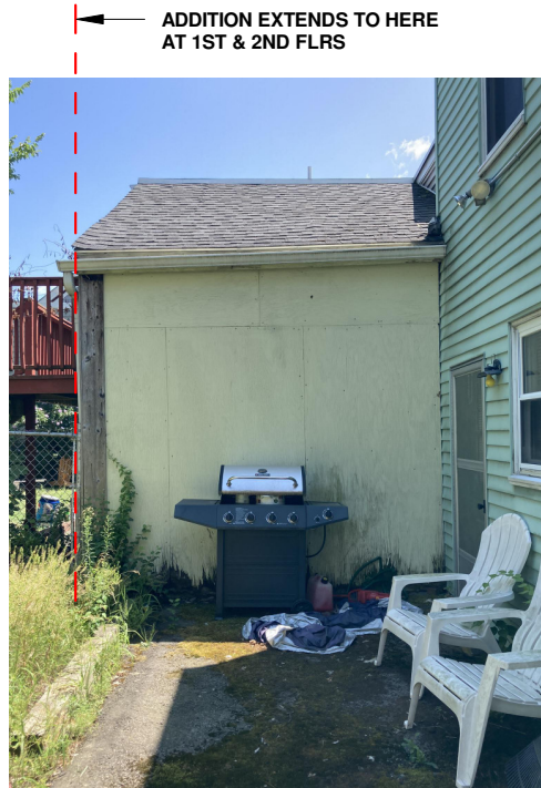
REAR YARD LOOKING AT #89 RIGHT SIDE NEIGHBOR
