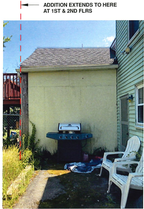
REAR YARD LOOKING AT #89 RIGHT SIDE NEIGHBOR
