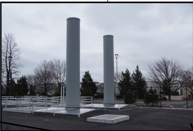
North Dorchester Bay Odor Control/Ventilation Facility
