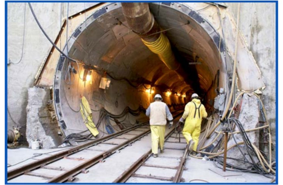
North Dorchester Bay Storage Tunnel
