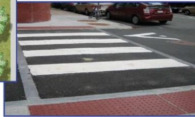
Curb Extensions & Ramps [for accessibility]
