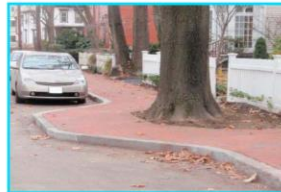
New Sidewalks [brick & concrete]
