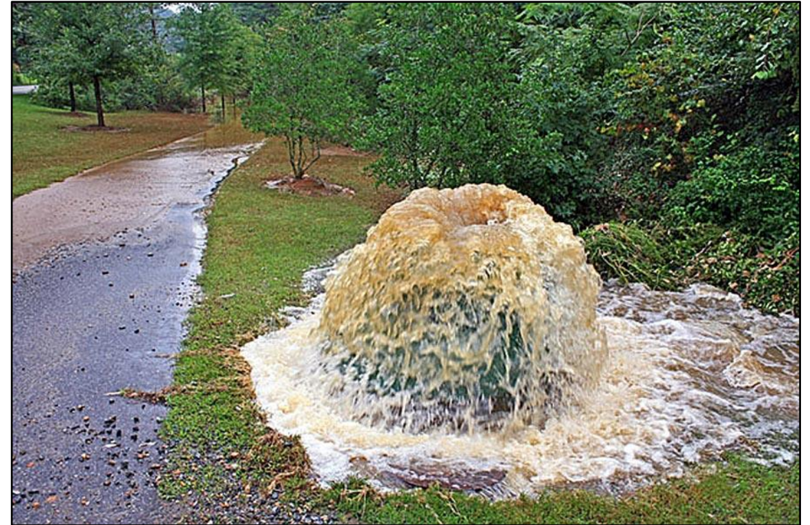
Sanitary Sewer Overflows (SSOs) release sewage in neighborhoods and can contribute to local flooding.
