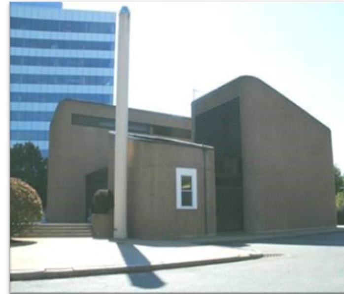
Prison Point CSO Facility
