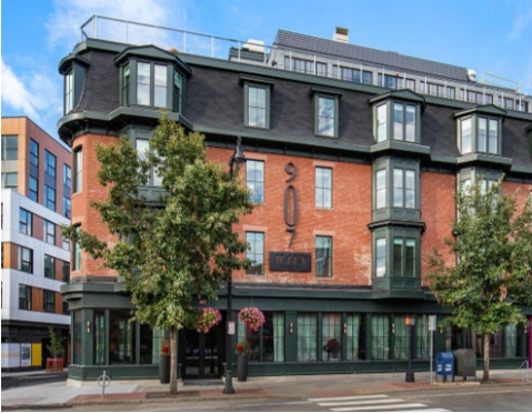
907 Main Street Hotel renovation/addition – built
