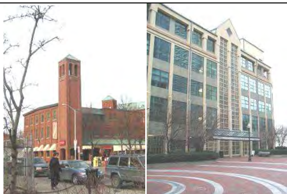
Existing buildings in IB District
