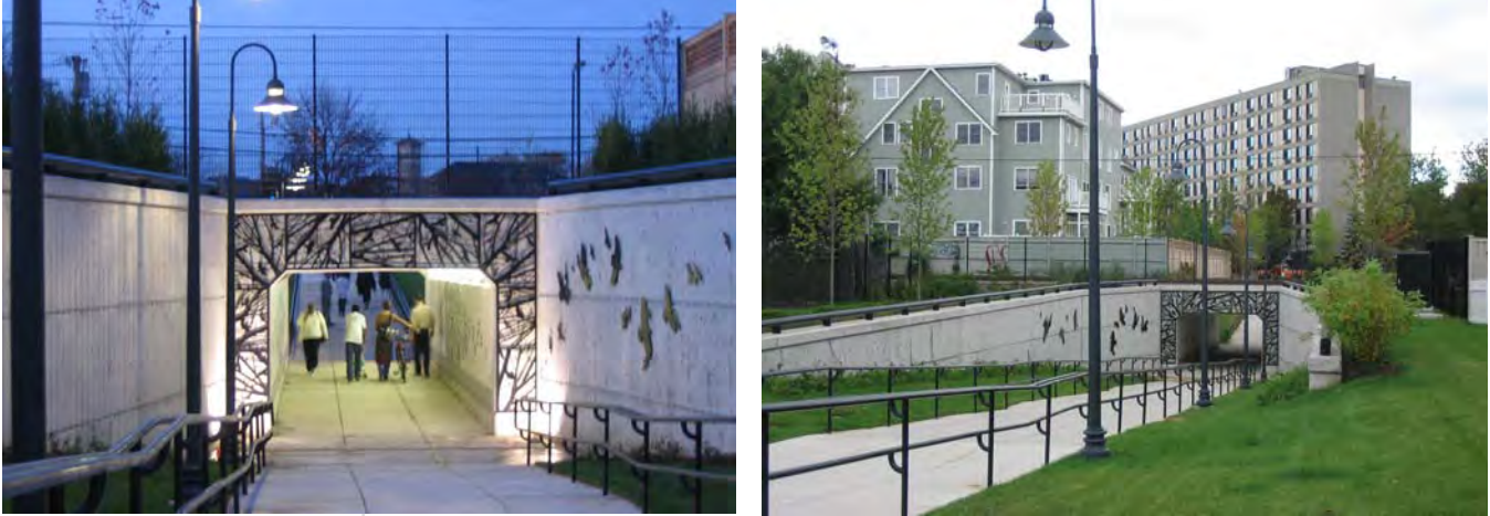
Figure 4 : Post Construction Photos
