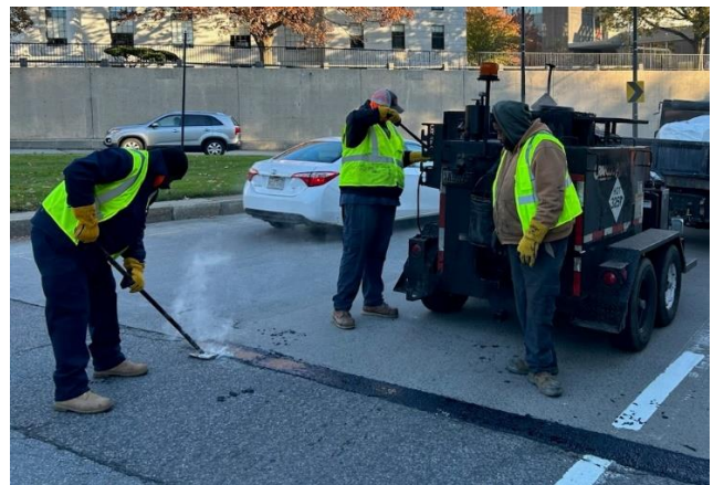
Repairing street in Harvard Square
