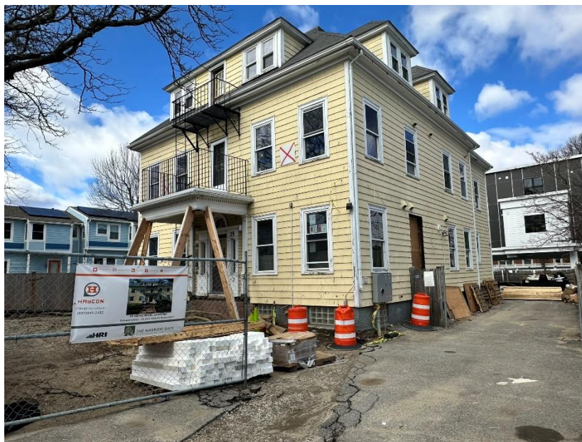
Renovations underway at 35 Harvey Street
