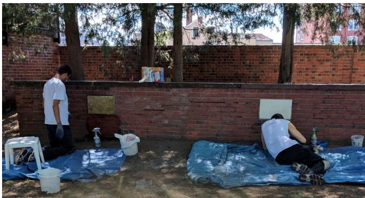
Old Burying Ground in Harvard Square – Tomb Repointing (left) & Headstone Mending (right)
