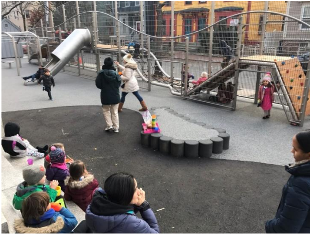
Amigos School Playground Renovation
