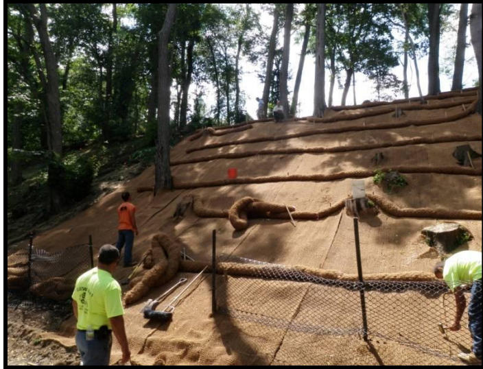
Glacken Slope Stabilization Project Under Construction View from Perimeter Road
