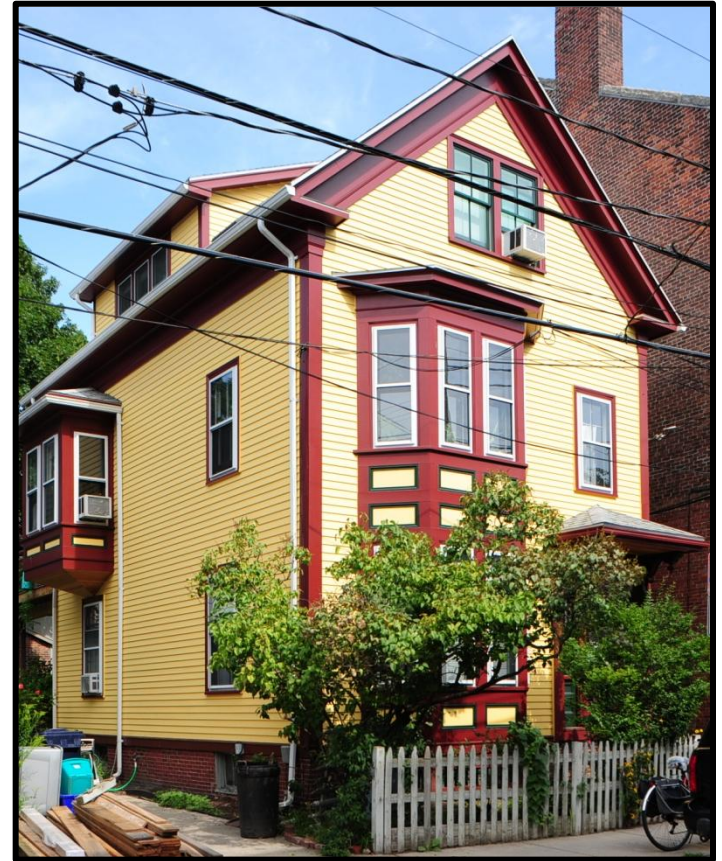
CPA-funded affordable housing projects enhance Cambridge neighborhoods
