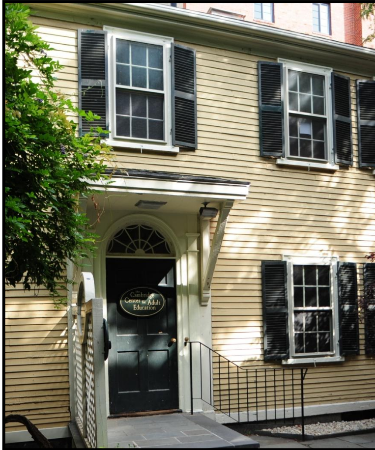
A Preservation Grant enabled the Cambridge Center for Adult Education to completely restore the exterior of the historic Blacksmith House.
