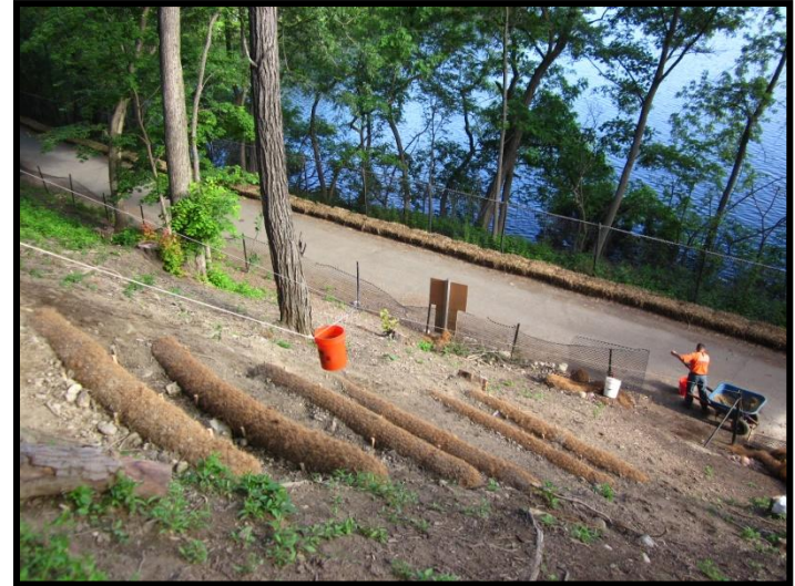
Glacken Slope Stabilization Project Under Construction View from Top of Slope
