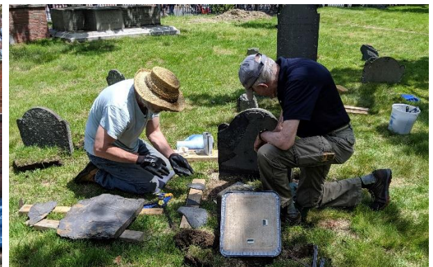
Old Burying Ground in Harvard Square – Tomb Repointing (left) & Headstone Mending (right)
