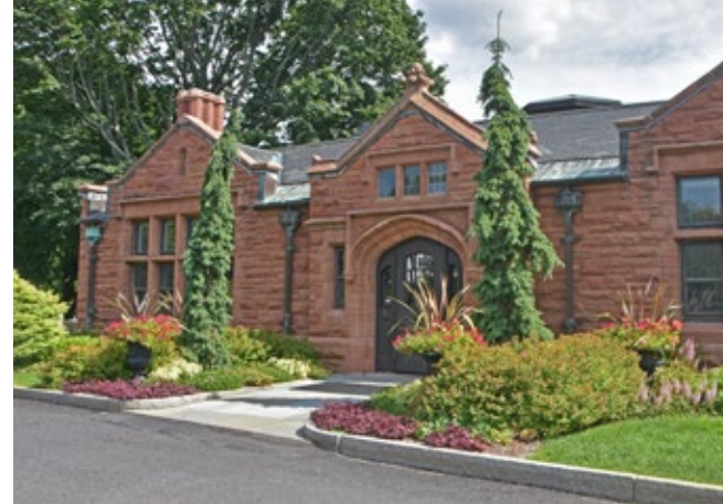
Mt. Auburn's Admin Building greets visitors with intense planting
