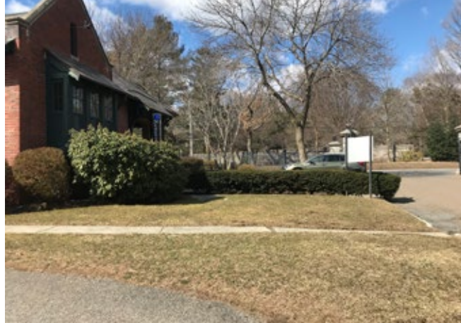
Frontage of Admin building is in need of landscape improvements
