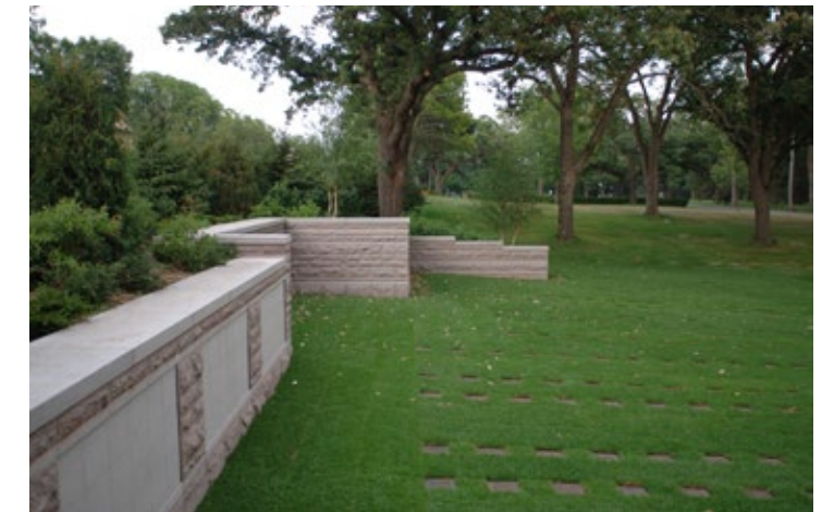
Figure 71. Retaining wall columbarium at Lakewood Cemetery, Minneapolis, MN.
