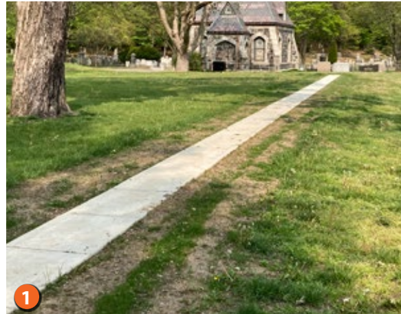
1 Latest infill area adjacent to the Chapel - foundation for headstones has been installed.
