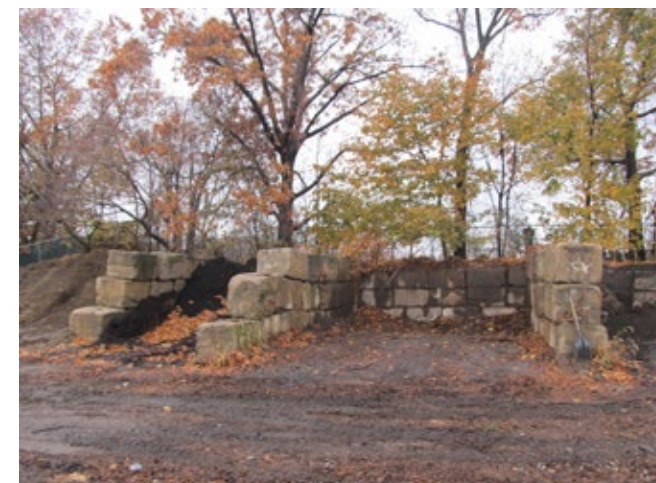
Materials Storage Yard is deteriorated and unkempt.
