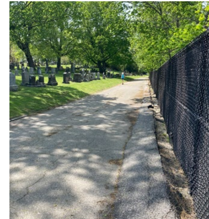
Figure 27. Asphalt berm along Meadow Avenue / BB&N property line.
