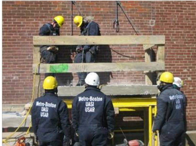
Shoring, stabilization, and breaching
