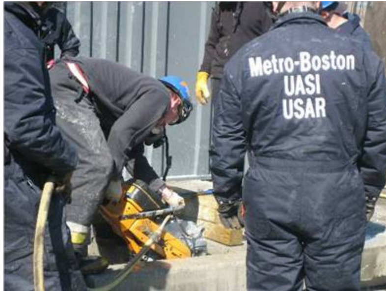
Concrete cutting saw station
