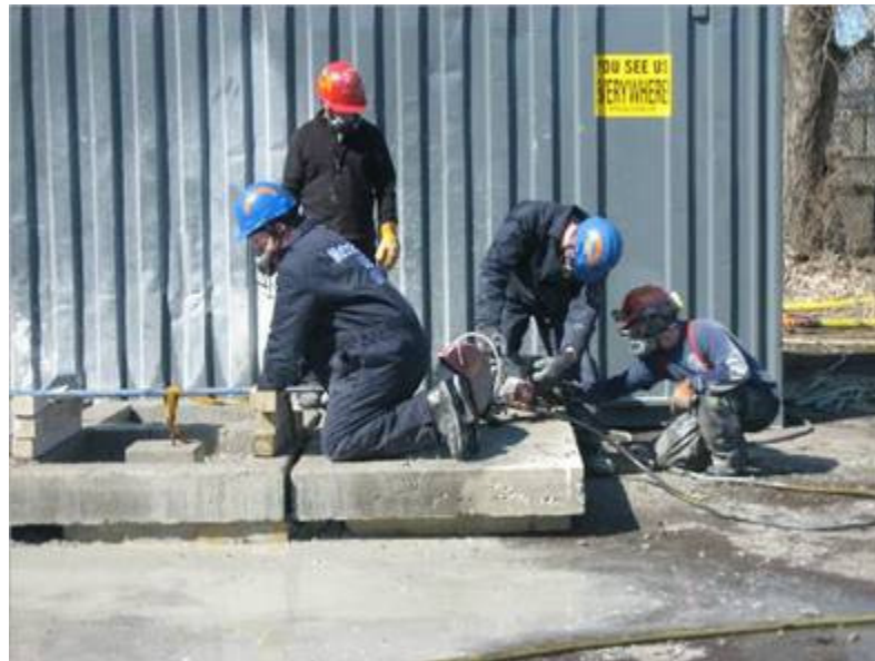
Concrete slab breaching station
