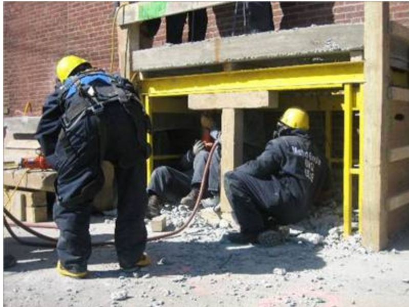
Pneumatic jack-hammer for concrete breaching
