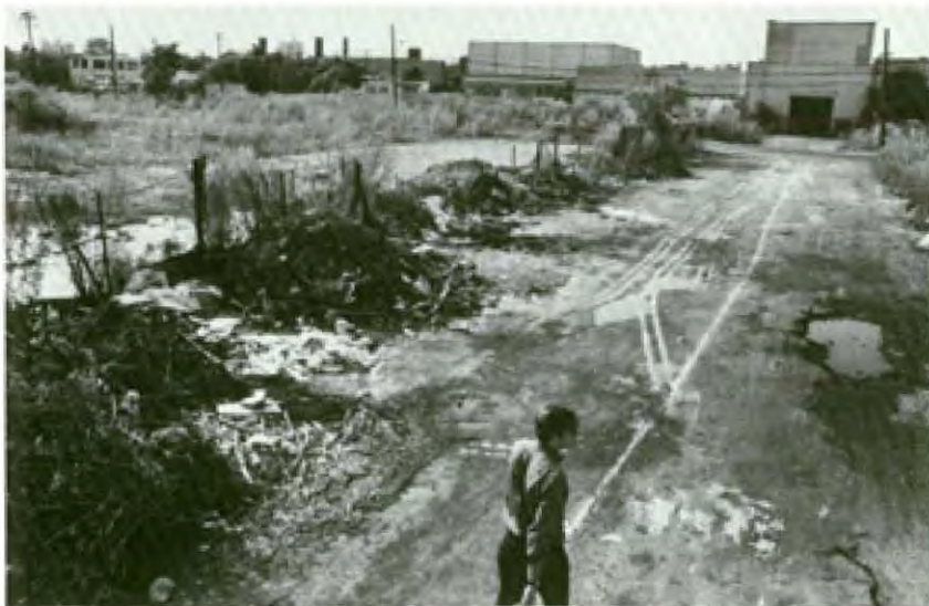
In the early 1970's, many of the Simplex Wire and Cable Company's buildings were razed, leaving acres of vacant land.
