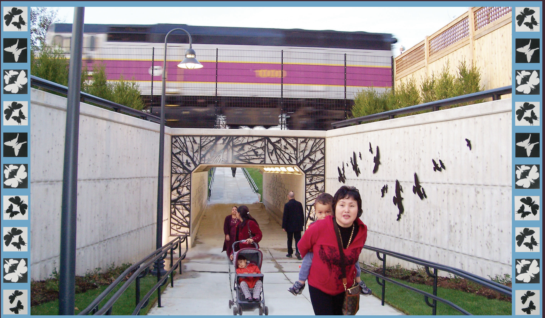
NEWLY COMPLETED YERXA ROAD UNDERPASS
