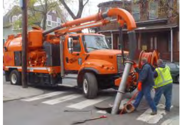
DPW crews work on sewer maintenance
