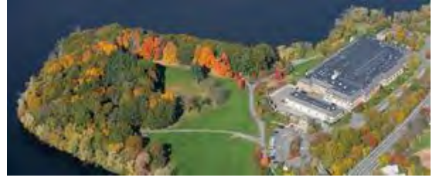
Aerial view of Cambridge Water Department
