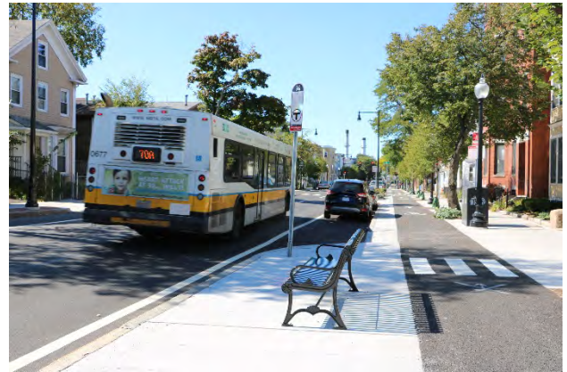
The separated cycle track on Western Avenue protects cyclists from parked and moving vehicles.
