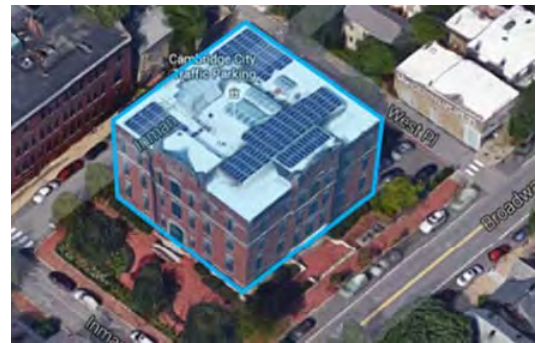
Energy reduction projects include comprehensive evaluations of building envelope to support efficiency projects.
