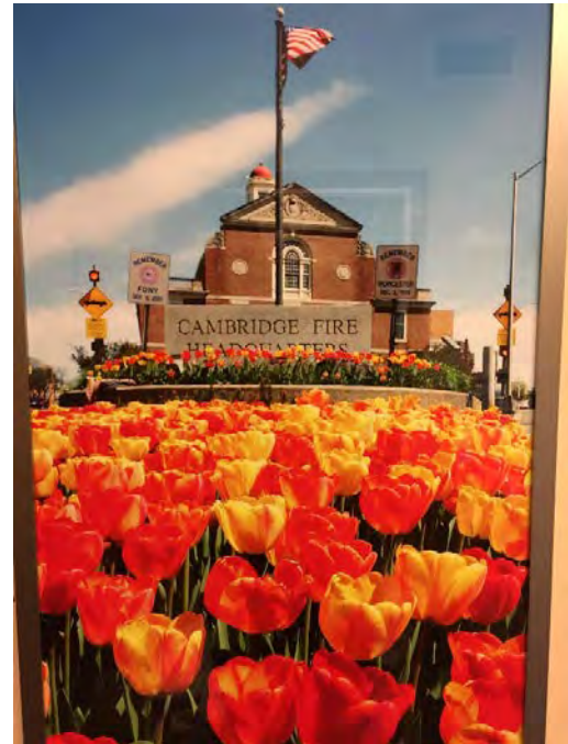
Fire Headquarters, built in 1934, houses Fire Administration, Engine One, Ladder One, Rescue One, Hazmat One, the Dive Rescue vehicle, and the Division Three SUV.
