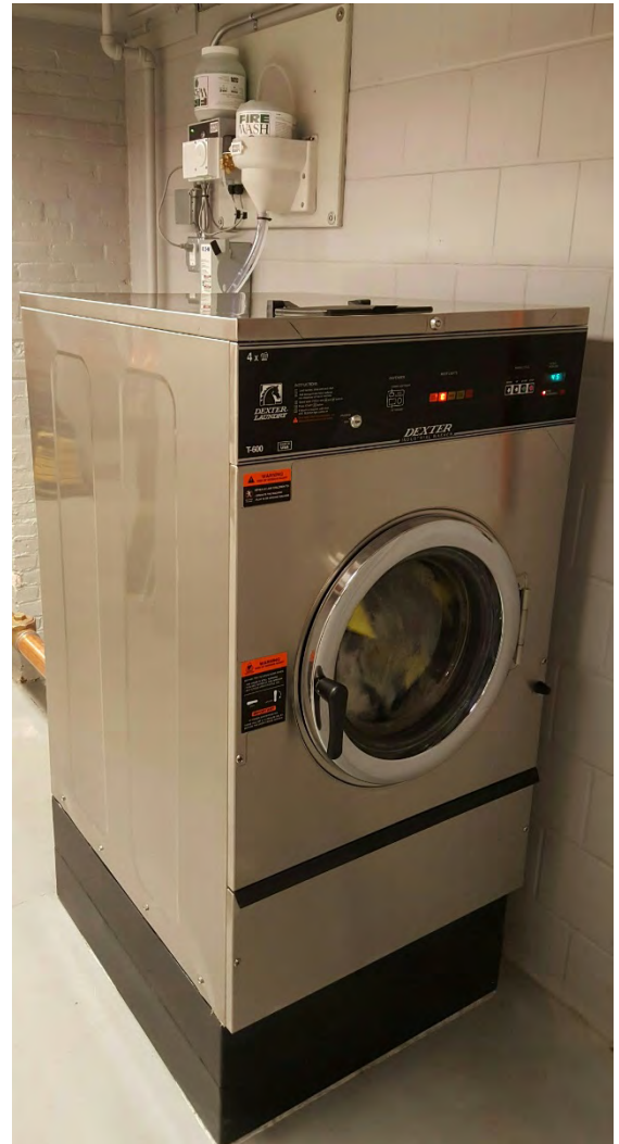
Firefighting gear washers have been installed in three fire stations and will soon be installed in a fourth. Products of combustion contain carcinogens that can permeate protective clothing, so CFD personnel are encouraged to wash their gear after each exposure.
