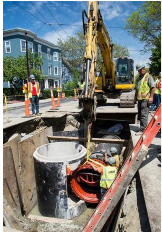
Sewer replacement work
