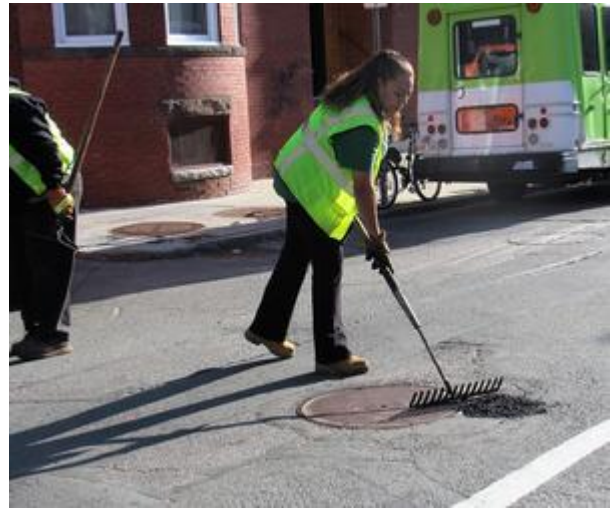
Repairing a pothole
