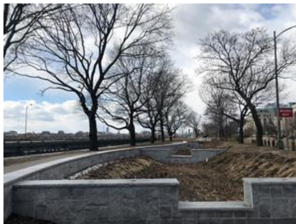
The Longfellow Bridge Project's subsurface gravel wetland
