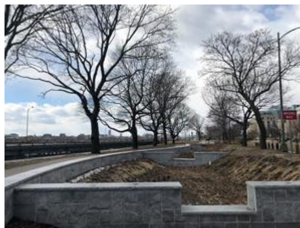
The Longfellow Bridge Project's subsurface gravel wetland
