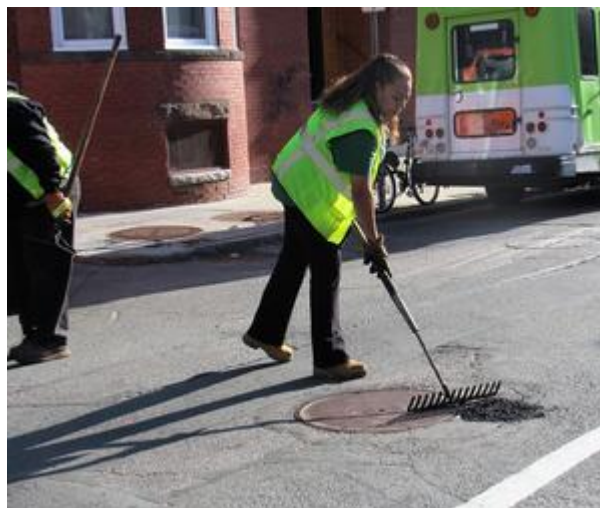
Repairing a pothole
