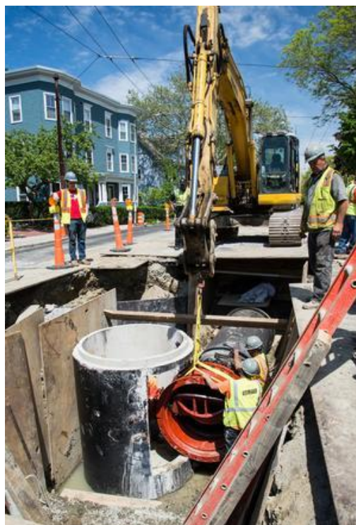
Sewer replacement work
