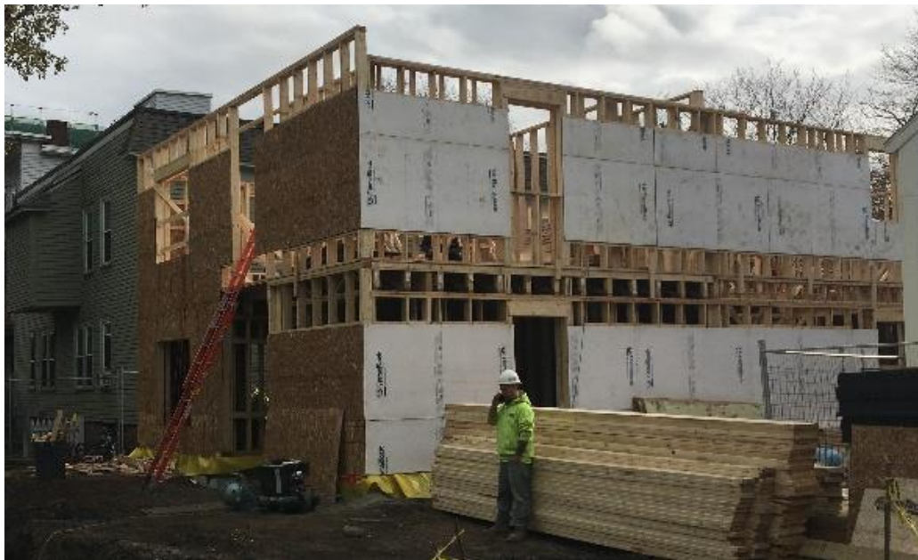
Construction is underway on 23 new affordable rental units in the Port.
