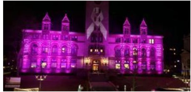
Updated City Hall LED lighting system
