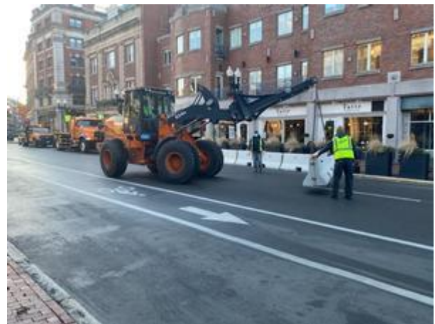
Installing barriers to facilitate outdoor dining in Harvard Square
