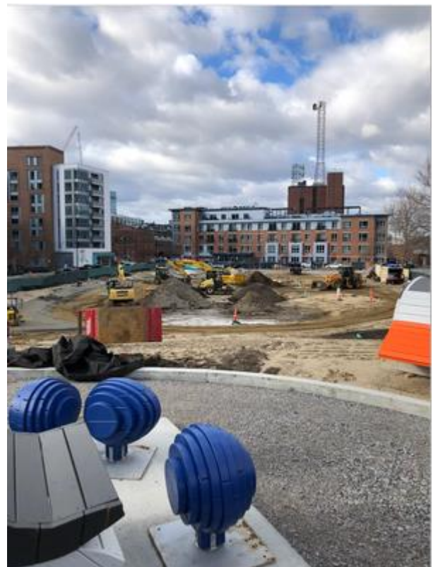
Construction at Timothy J. Toomey, Jr. Park
