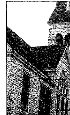
NORTH SIDE ROOF, GUTTERS, DOWNSPOUT, CHEEK WALLS OF CROSS GABLE
