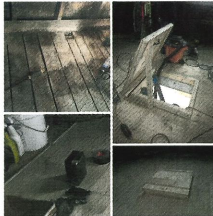
Repairs In Spire (Before/After)
