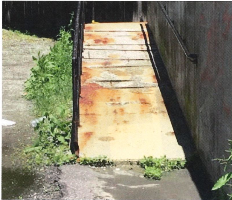
EXISTING REAR HANDICAP RAMP
