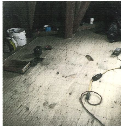
New Floor Boards
