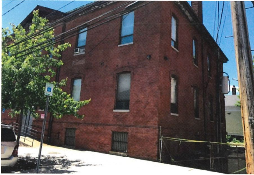
EXISTING FRONT FACING RIGHT CORNER
