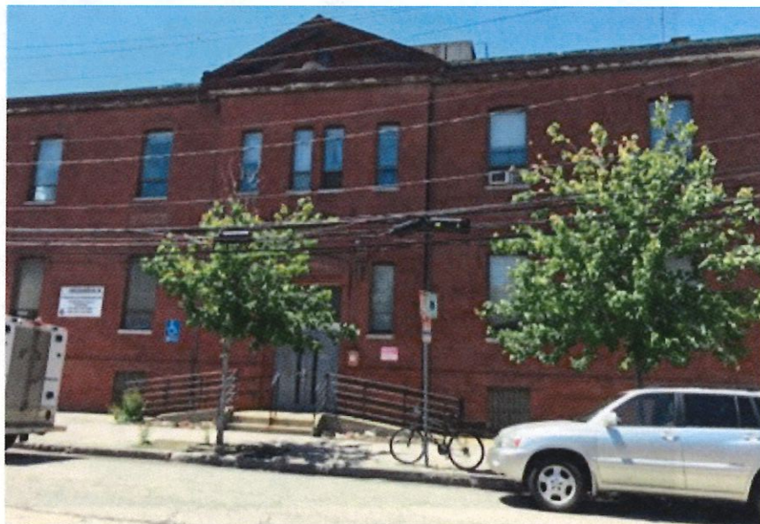
EXISTING FRONT OF BUILDING
