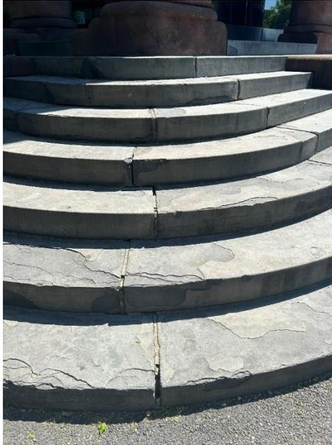
The Cambridge Public Library is requesting funding for the repair of the original 1888 slate and brownstone entry stairs located at the southwest corner of the building. They have weathered badly over the last 15 years and much of the mortar has failed leaving the original stone susceptible to water infiltration and freeze thaw damage.
