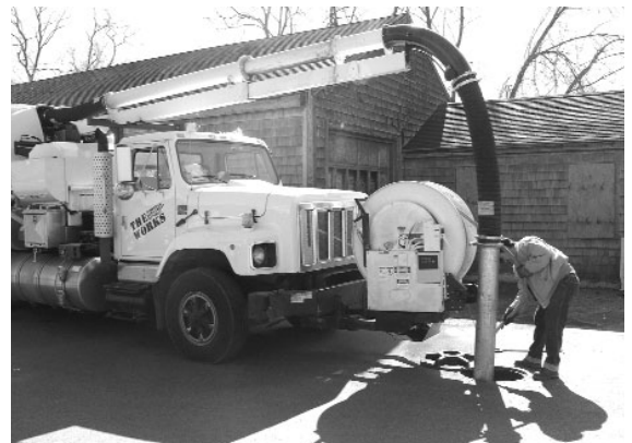
Sewer Division employee operating the Vactor Truck near Fresh Pond.
