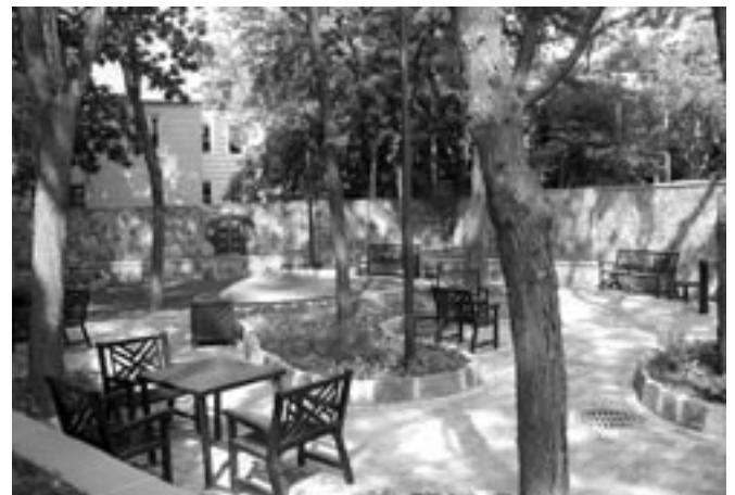
Renovations to the Franklin Street Park included new lighting and site amenities, tree work, and improved access.
