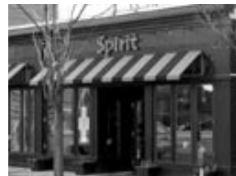
Facade improvements, such as this one at 2046 Mass. Ave. in North Cambridge, were completed throughout the City to enhance the character of the retail environment.
