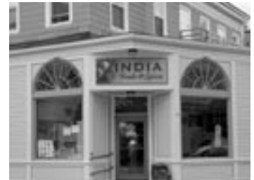
Façade improvements at 80 River Street were completed this year as part of the City's Façade Improvement Program, which provides matching grant funds to upgrade commercial storefronts.
