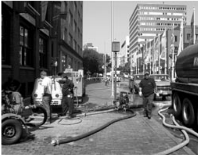
CWD crew repairing a leak to a 12" water main on Broadway.
