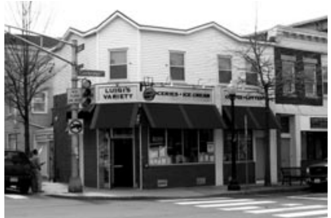
Storefront improvements at 520 Cambridge Street were completed this year as part of the City's Façade Improvement Program.
