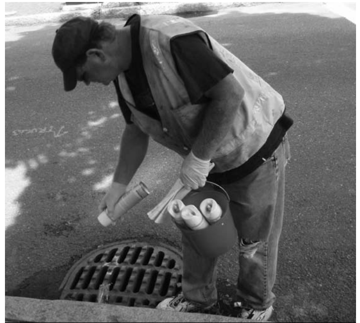
The Sewer Division coordinated the City's program to control mosquito breeding at public owned catch basins, ensuring that each of the City's 4,000 catch basins were treated twice during the summer of 2006 to prevent the development of adult mosquitoes and reduce the risk of West Nile Virus. [Photo Credit: Wendy Robinson]
