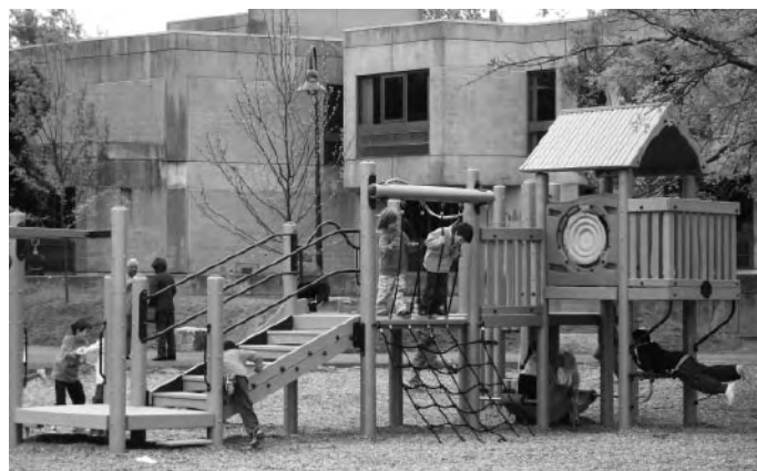
Renovations to the Father Callanan Playground at the Tobin School were completed this year, featuring a new play structure and swings for 5-12 year olds, an enclosed play area for younger children, new basketball courts, water features, and new paving, lighting and landscaping.
