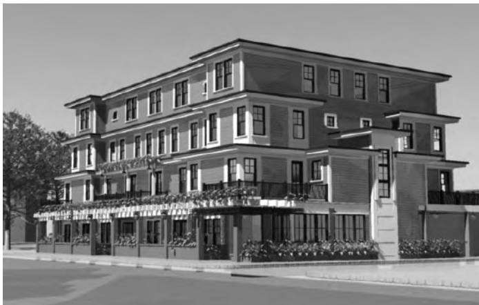
Construction began this year at 823 Main Street, where 10 units of affordable housing for first-time homebuyers will be built to LEED (Leadership in Energy & Environmental Design) standards using "green" construction methods. Boyes-Watson Architects
