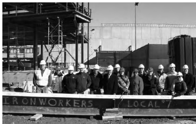
The Main Library project team, along with Library trustees, staff and members of the City administration celebrated the installation of the last iron beam on the new Main Library building.
