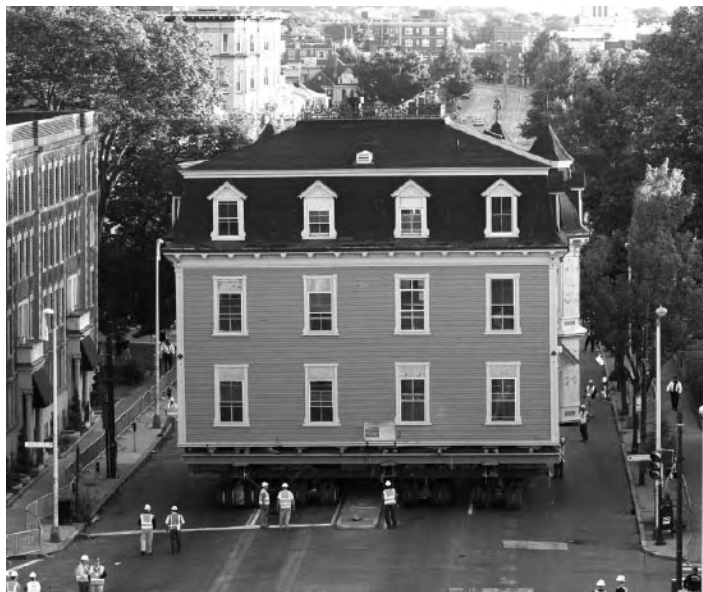
Harvard University complied with the CHC's request to move three Law School buildings on Mass. Ave. to a new site rather than demolish them. Pictured: One of the buildings, Harvard's Ukrainian Center (built in 1876 for Dr. Alden Keene), passes Everett Street on its journey north along Mass. Ave. toward Mellen St. Photo: Harvard Law School
