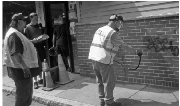
This year, DPW worked with the Police Department to continue a graffiti removal program with a graffiti steam cleaning and power washing machine that was instrumental in the completion of over 100 graffiti removal jobs.
