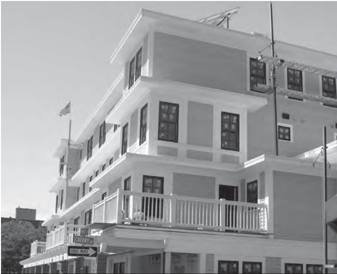
At 823 Main Street in Area IV, construction of 10 affordable condominiums for first-time homebuyers is almost complete.
