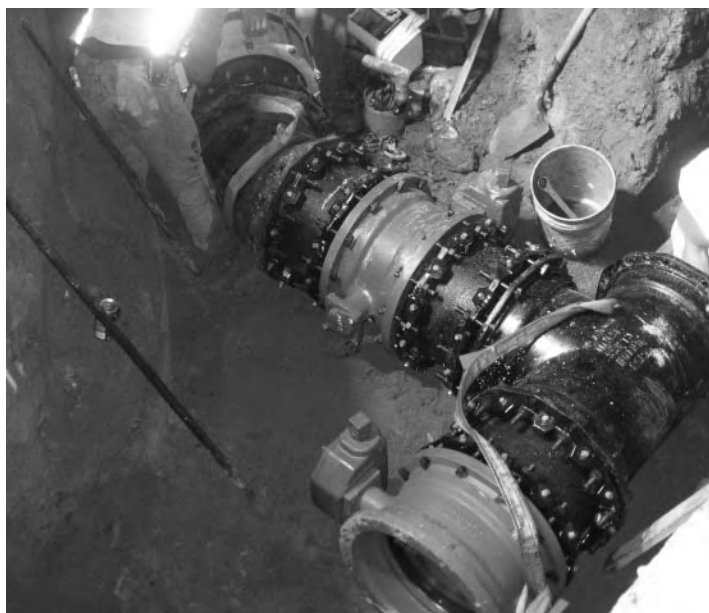
New 16" water main and valves on Concord Avenue.
