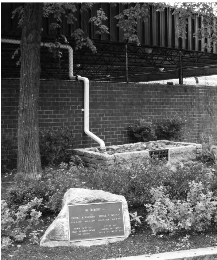
A new rain garden at the DPW Frazier Building helps manage stormwater and reduces pollutants going directly to our water systems.
