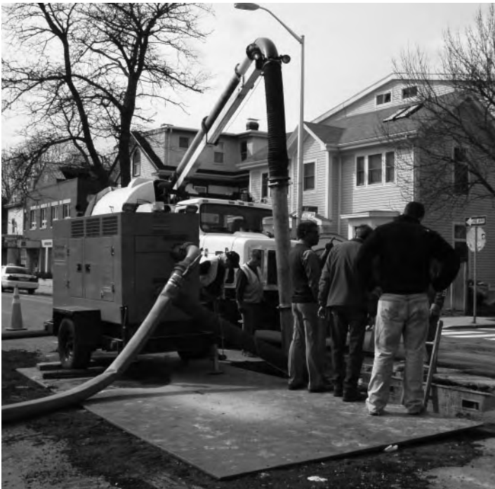
Streets and Sewer Maintenance staff conducting utility investigations on Western Avenue.
