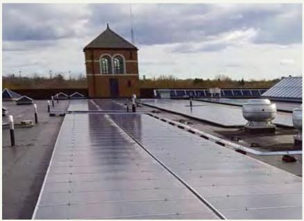
The new Dr. Martin Luther King, Jr. School complex targets Net Zero energy consumption, saving energy through proper orientation, pervasive natural light in most spaces, and a high-performance roof with over 1,600 photovoltaic (solar) panels, which are estimated to provide 47% of the building's required energy. It also offsets energy demands through the use of photovoltaic panels mounted on the roof and south-facing facades.
