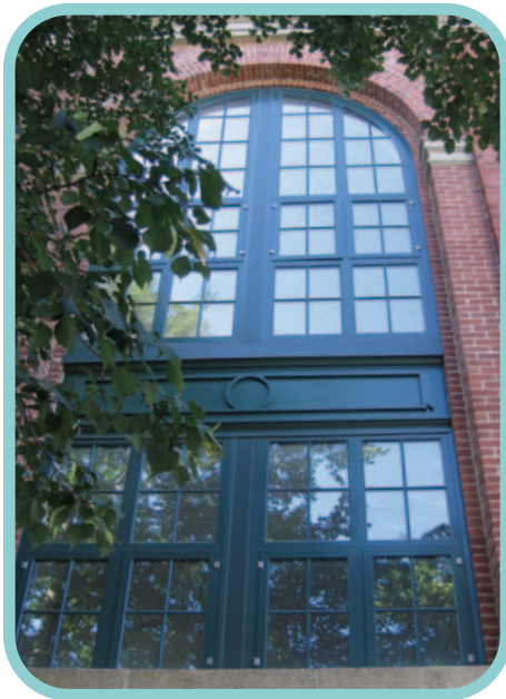
Photo, Opposite Page: A side view of the former switch house in Riverside that was redeveloped as permanently affordable housing.
