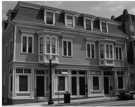
Cascap completed rehab of six affordable rental units on Cambridge St.
