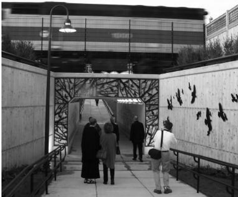
A commuter rail train passes above while pedestrians safely cross below in the recently completed underpass. Artist Randall Thurston created the striking design for the double entrance and interior tile walls.
