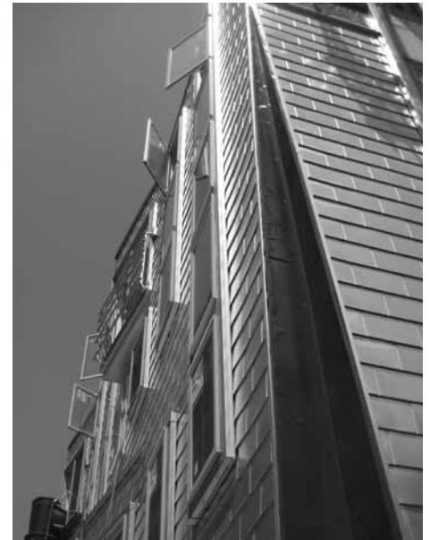
Cascap is completing 24 affordable units on Harvard Street. A former print shop, the site has been transformed by a modern building constructed with sustainable materials and energy efficient features. New owners will benefit from the recently completed Greene • Rose Heritage Park.
